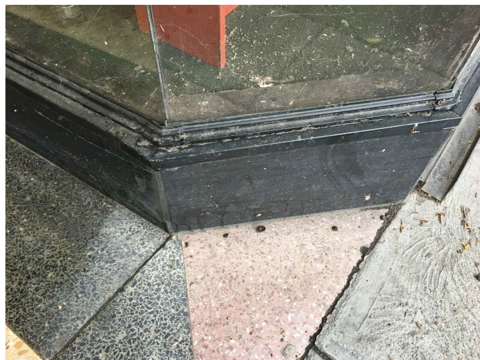
EXISTING METAL STOREFRONT AND CURB
