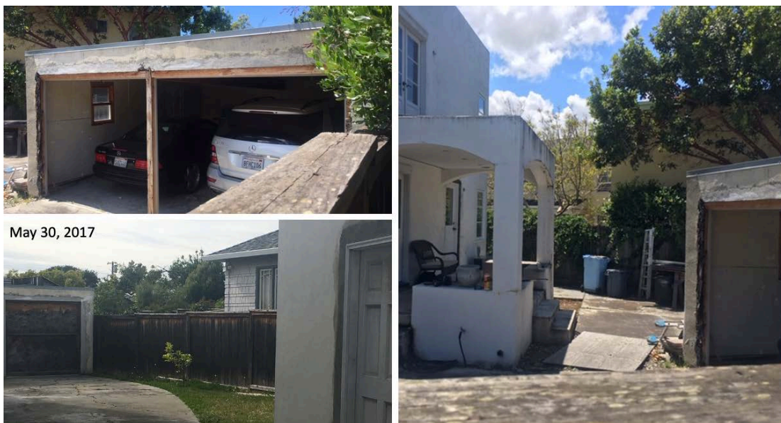
Figure 5. The upper left and right photo were taken May 18, 2020 and would be the views from our daughter's window if the hedge was not there. The lower left photo was taken May 30, 2017 (from the sidewalk), and demonstrate the disrepair of the Appellant's property that has existed since we moved in.
