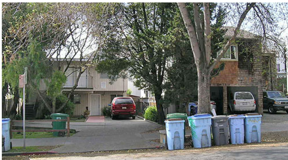
Figure 88. 2402–2404 (r) & 2406 Dana Street
