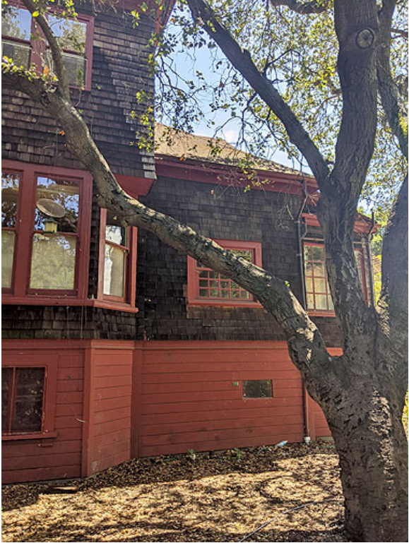
Figure 20. West façade, southern end
