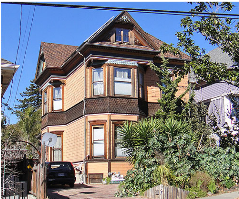
Figure 45. Langdon & Carrie Smith House (1894), 2155 Vine Street
