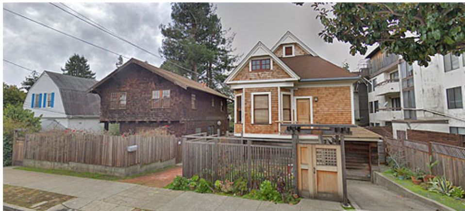
Figure 89. 1300 block of Bonita Avenue, west side (Google Street View)
