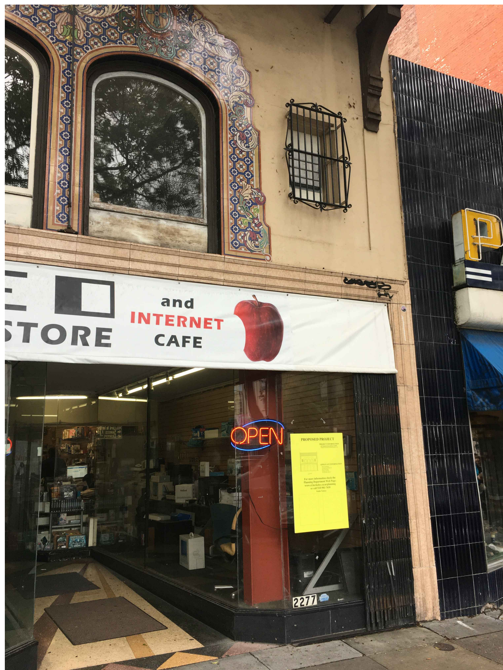
EXISTING GLASS AND METAL STOREFRONT
