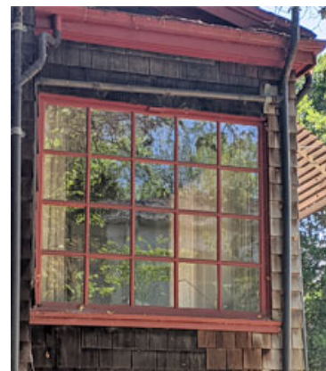
Figure 15. West-facing window in front porch
