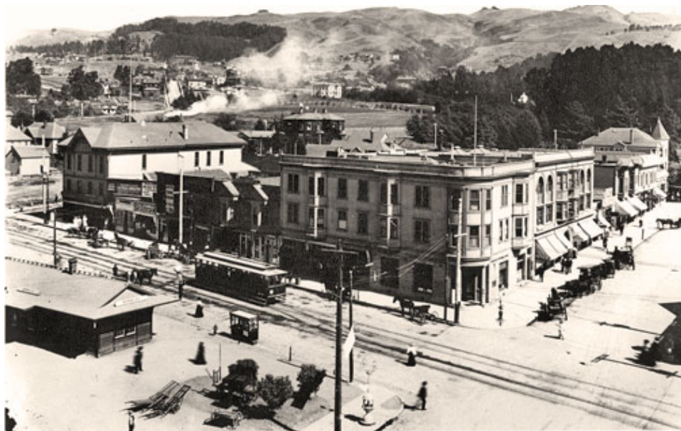
Figure 48. Odd Fellows' Hall (l) opposite Berkeley Station, c. 1906
