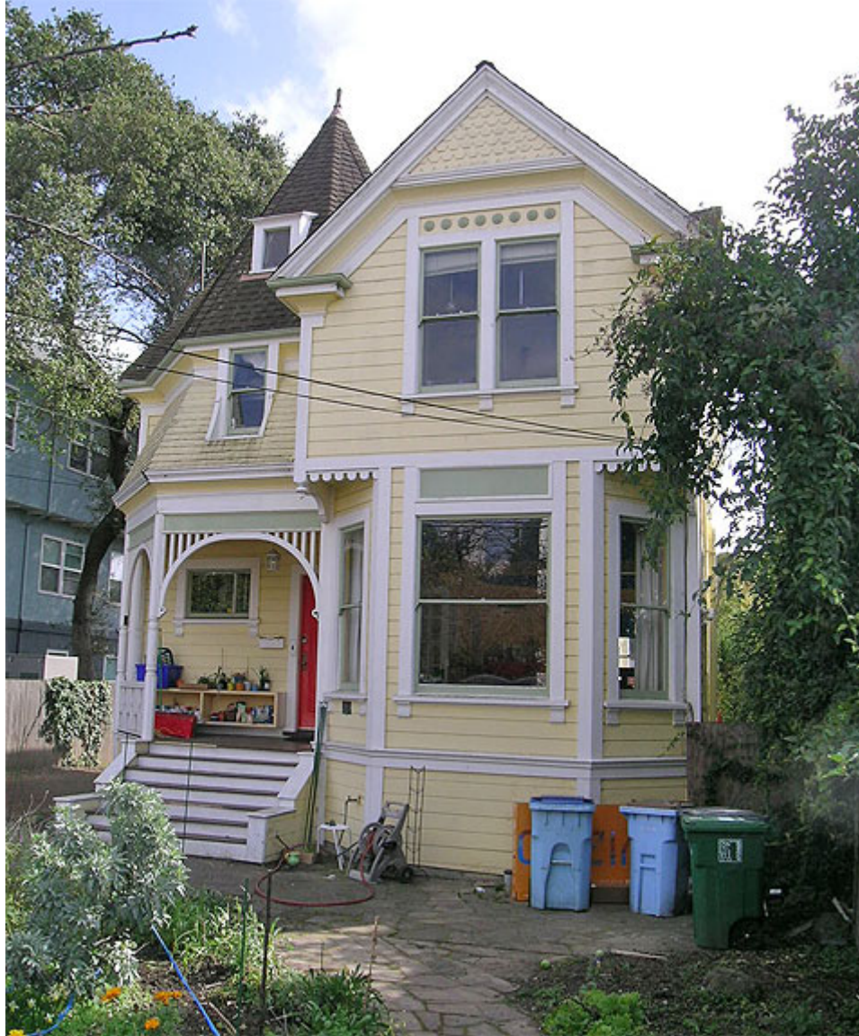
Figure 2. The Luttrell House, February 2020
