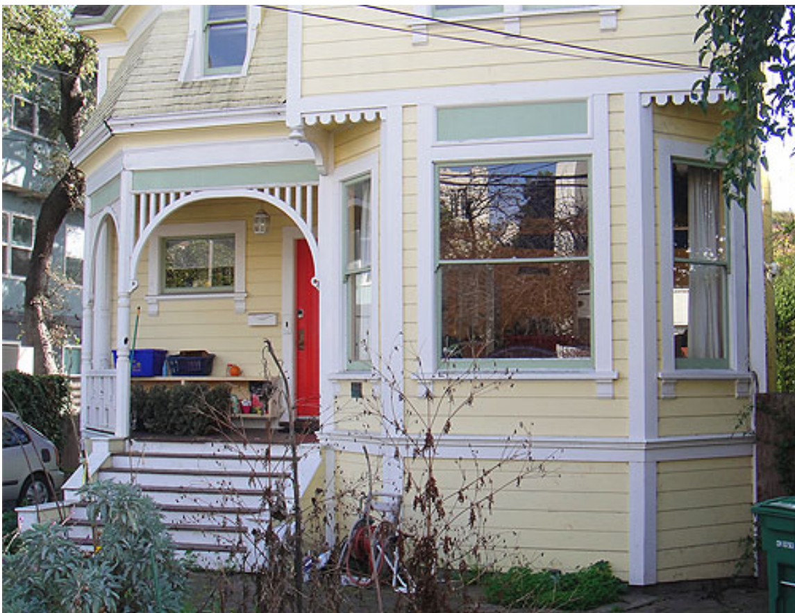
Figure 15. Ground floor, front façade
