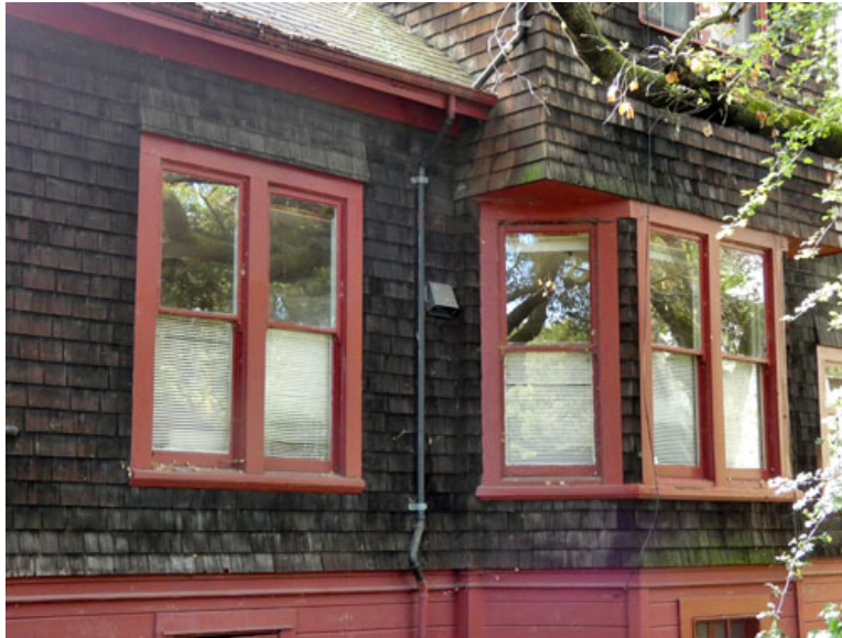
Figure 18. Windows on main level, west façade
