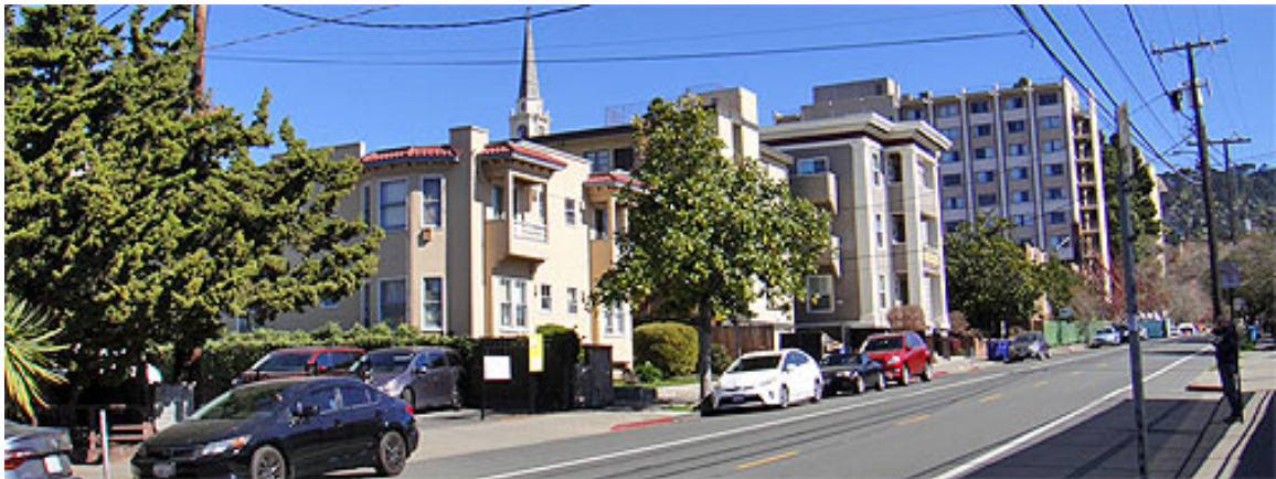
Figure 66. Channing Way, looking east
