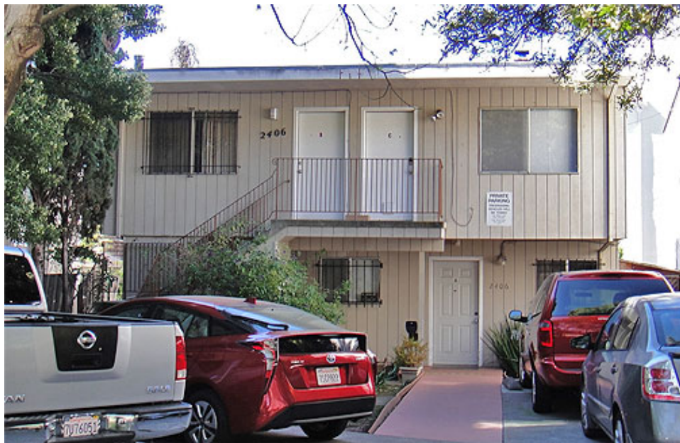
Figure 87. A 1975 triplex at 2406 Dana Street, 2020
