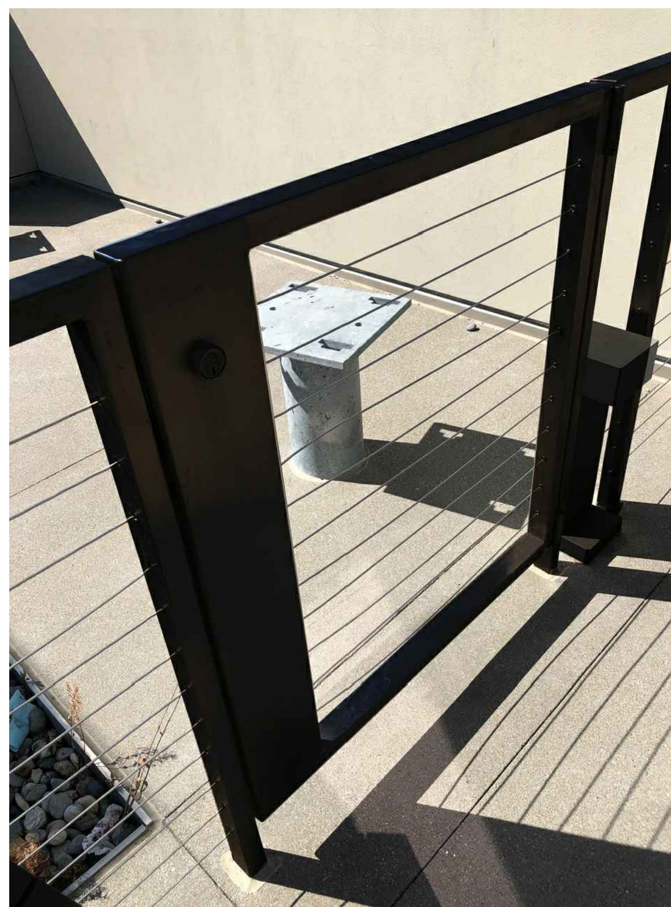
NEW ENTRY GATE WITH CABLE RAIL INFILL
