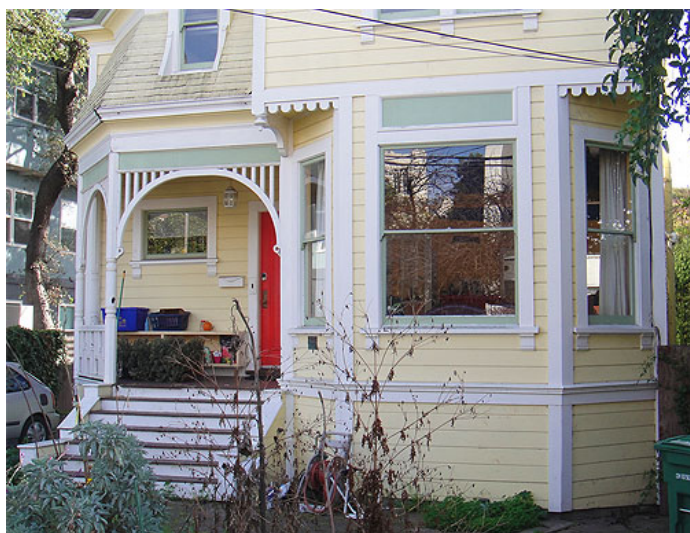
Figure 9. Rustic siding, Luttrell House
