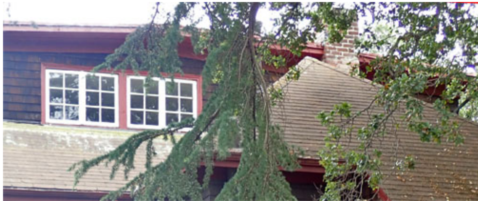
Figure 31. Brick chimney, north side
