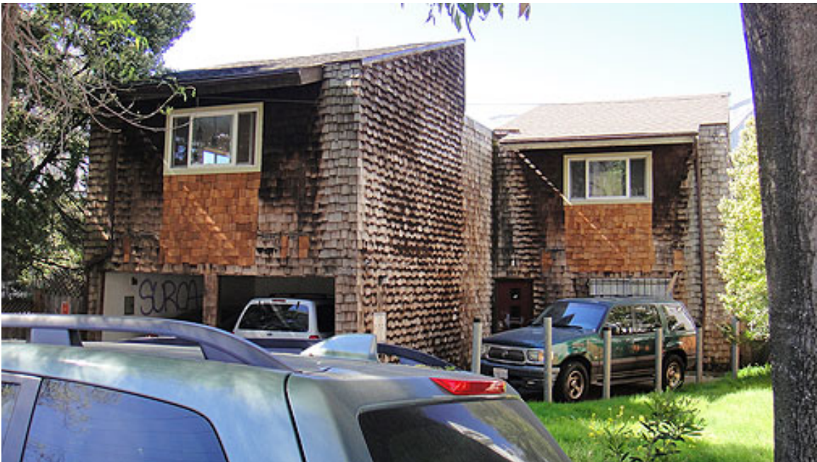
Figure 92. Townhouses at 2402–2404 Dana Street
