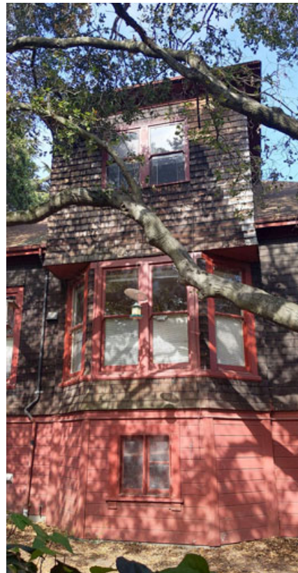
Figure 23. Bay window & second story, west façade
