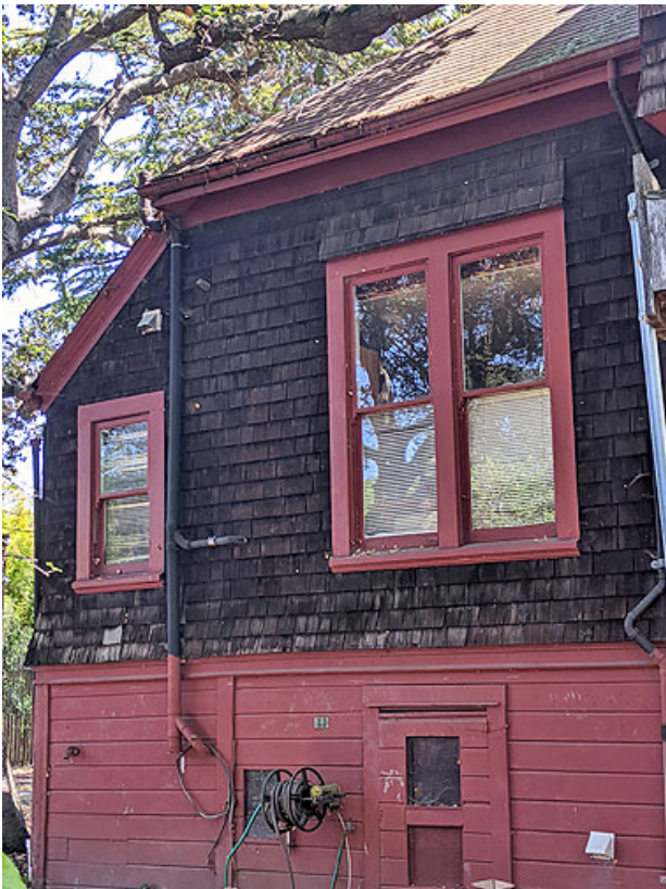
Figure 22. West façade toward the north
