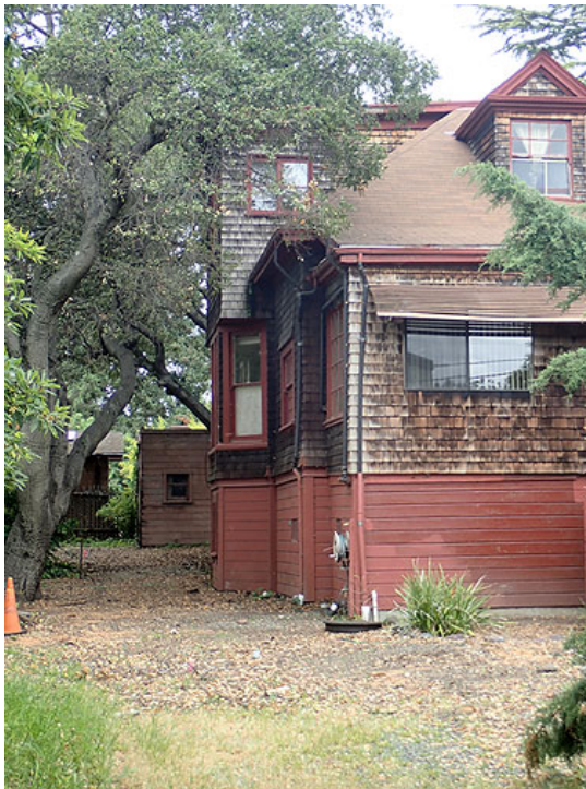
Figure 14. Enclosed porch, southwest corner
