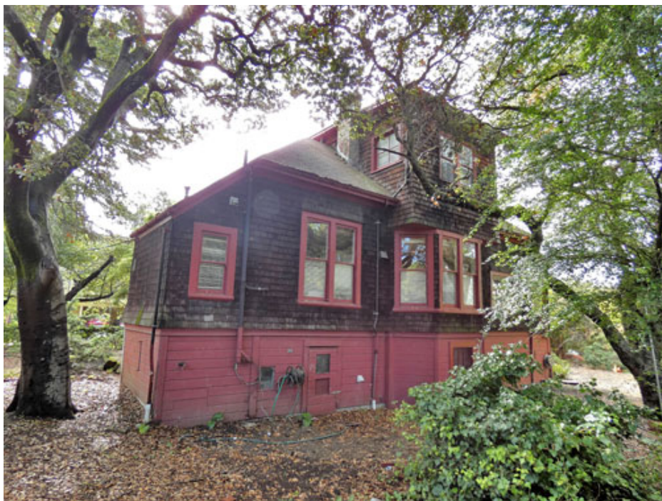
Figure 16. West façade, seen from the northwest
