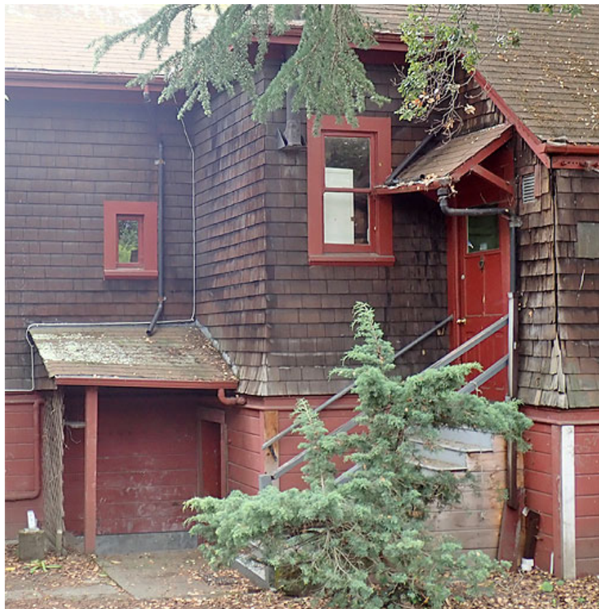
Figure 32. Cellar & service entrances
