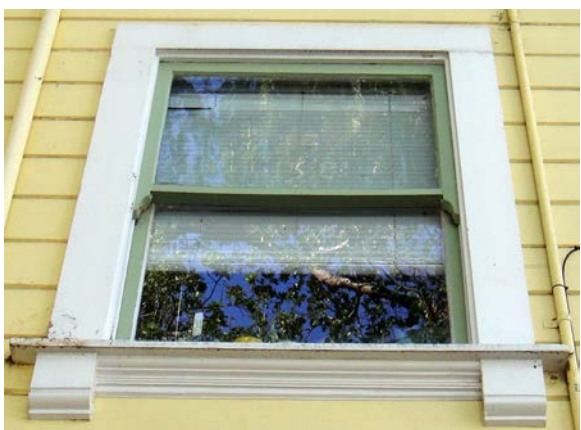
Figure 20. Mid-story window on east façade
