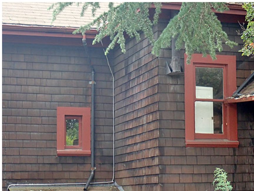
Figure 33. Windows, north façade
