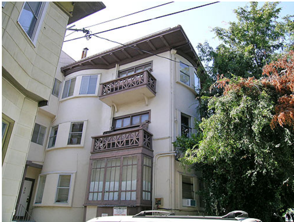
Figure 104. Balconies at 2410 Dana Street, 2007
