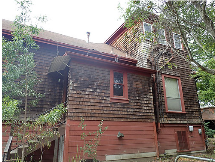
Figure 26. East façade, front & central sections
