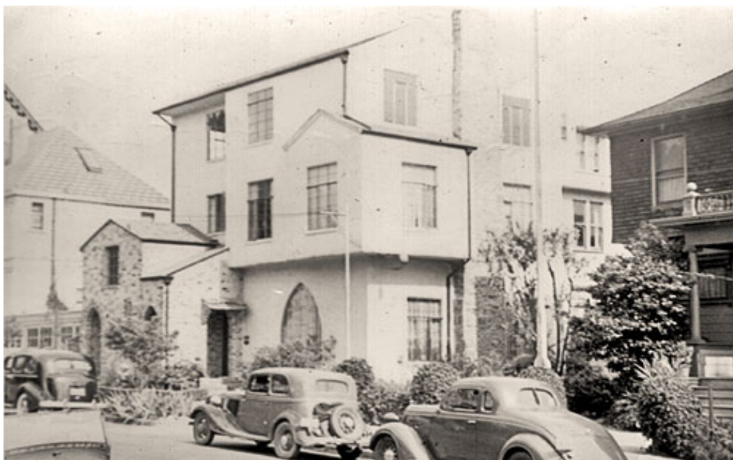
Figure 90. Francis Wood Apartments, 2336–38 Channing Way, in 1939 (Donogh)
