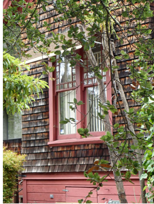
Figure 13. Windows in front wing
