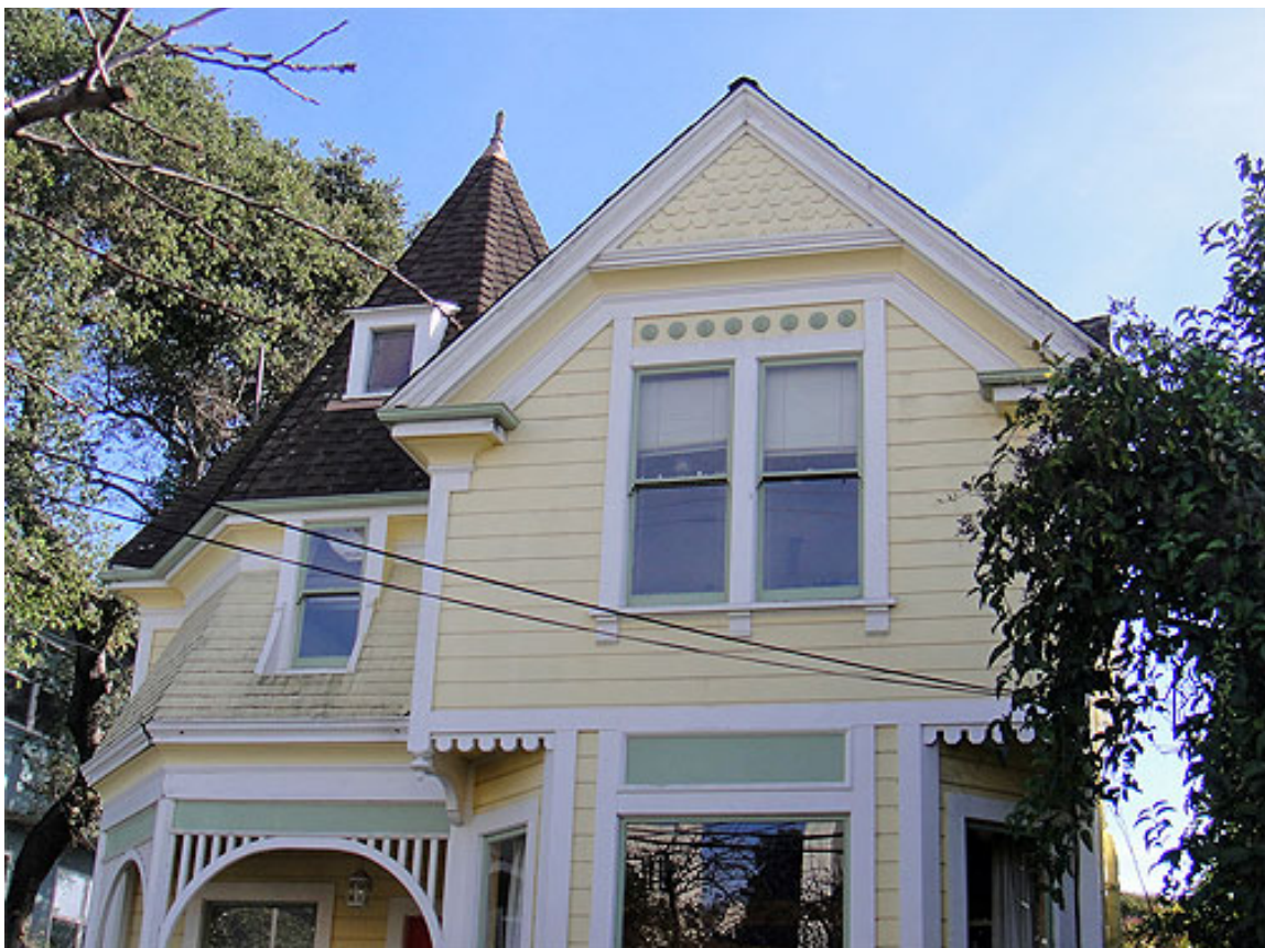
Figure 9. Upper floor, front façade
