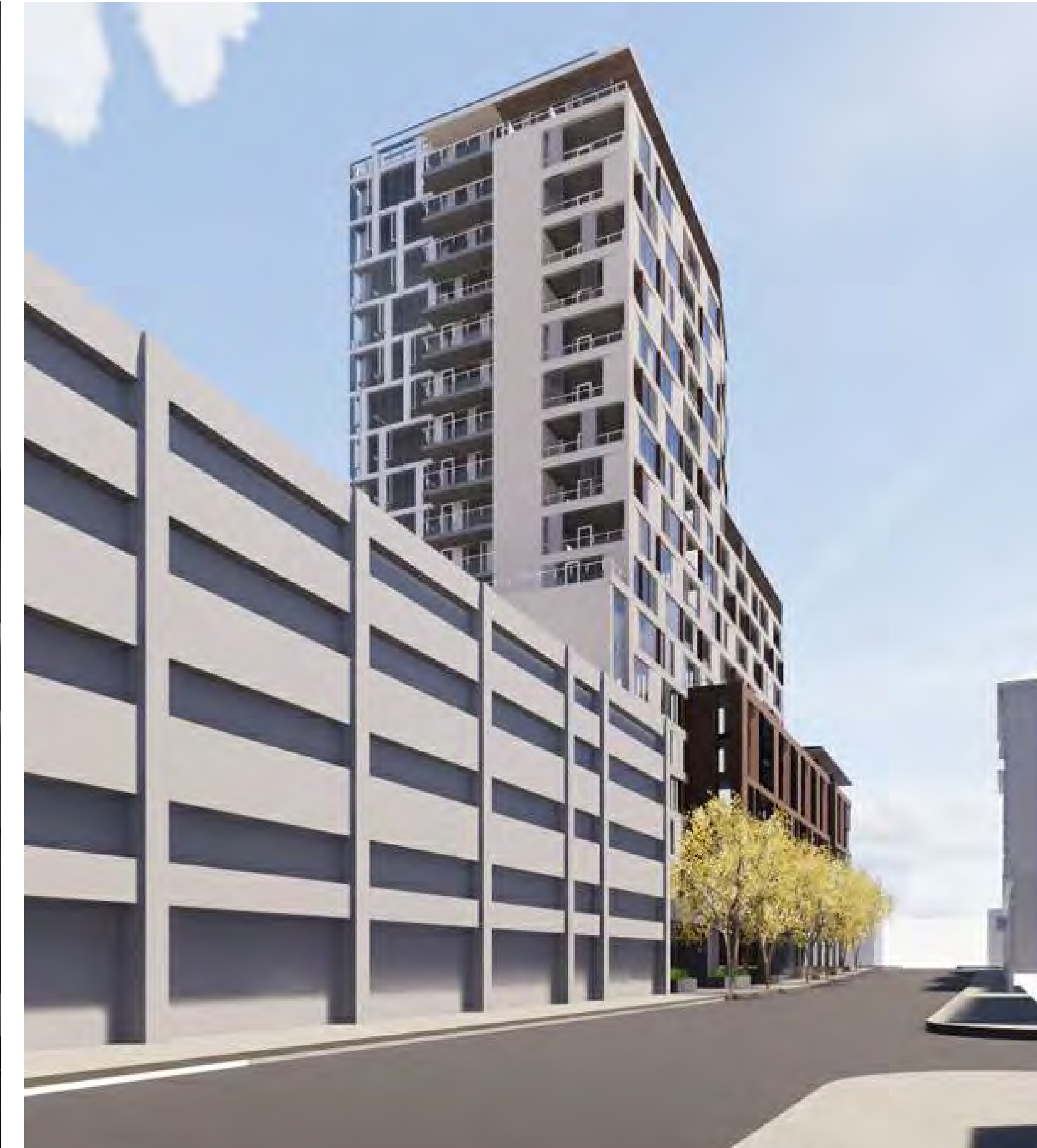
SOUTH WEST VIEW FROM ALLSTON WAY
