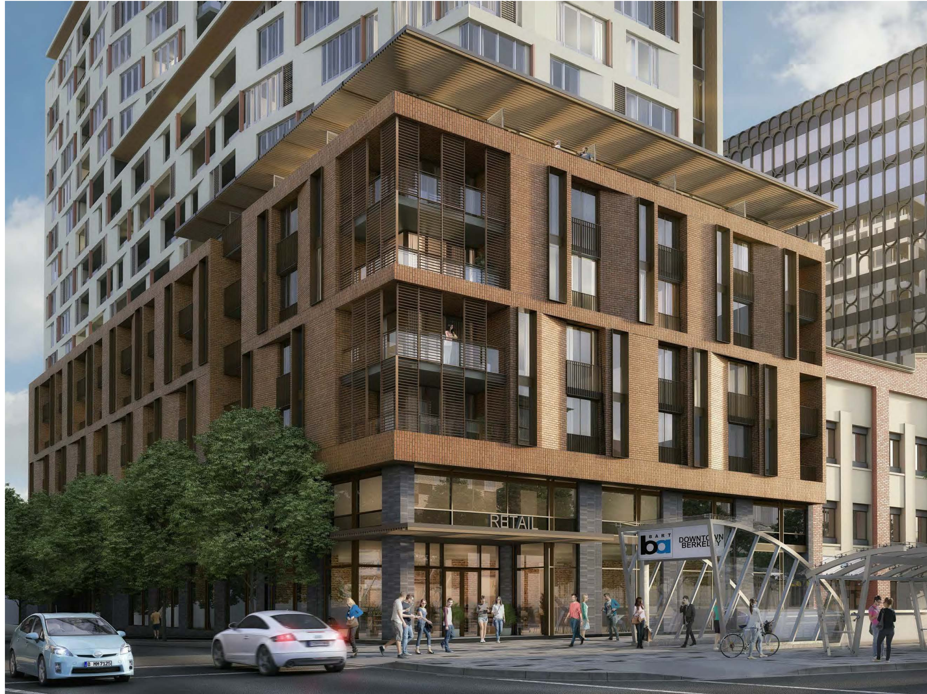
CLOSE UP VIEW FROM SHATTUCK AVENUE
