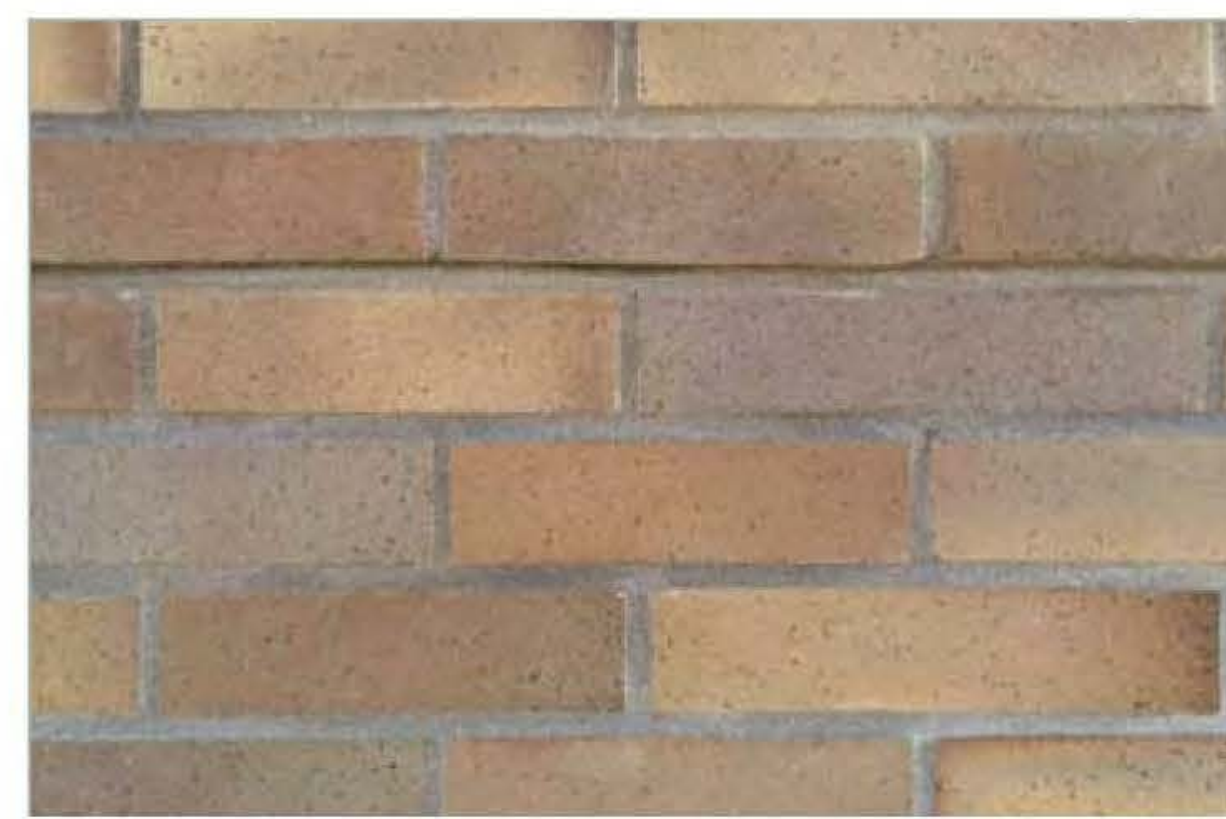
BRICK VENEER AT BUILDING BASE
