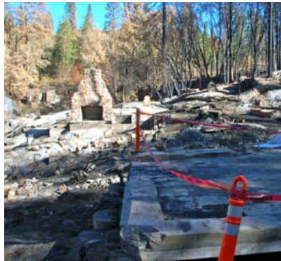
Dining Hall after fire (10/30/13)
