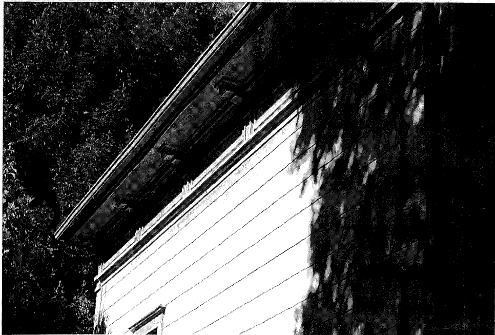
Figure 2. Bracketed eaves and band of paneling
