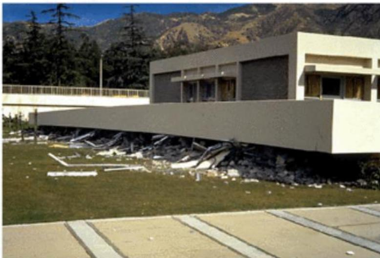
**Figure 1-1. 1971 San Fernando Earthquake, Olive Valley Hospital, was once two stories.** Source: World Housing Encyclopedia. [http://www.world-housing.net/uploads/101108\\_111\\_10.jpg](http://www.world-housing.net/uploads/101108_111_10.jpg)
