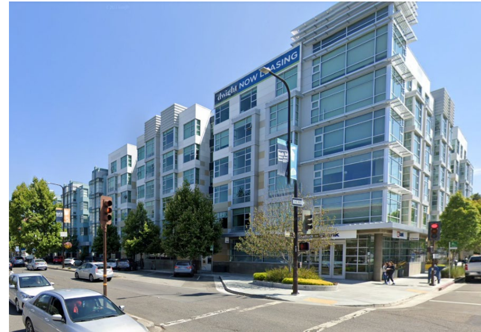
Building with major and minor breaks
