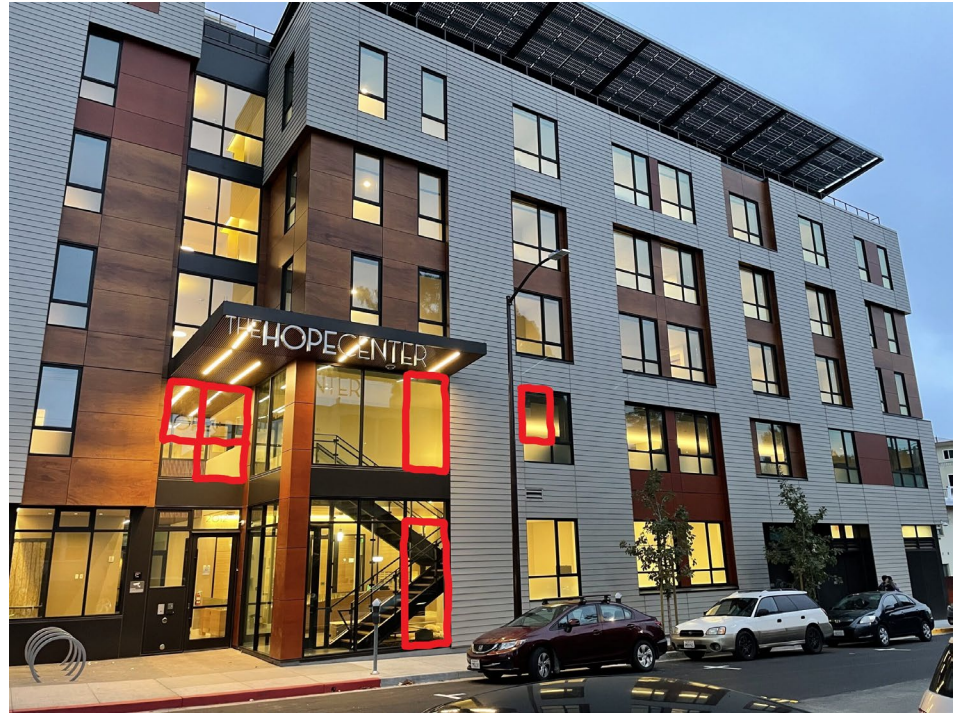
Berkeley Way affordable housing, Downtown (Source: Nibbi Brothers General Contractors)
