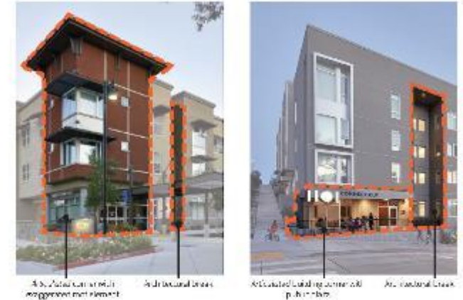
Fig. 3.7. Define corners and articulation with great detail, including an exaggerated cornice and a recessed sign from a structure below, on the building next to it. Add the building.
