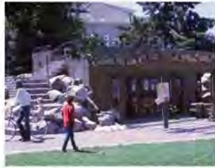
Original clubhouse with unpainted wood, roof terrace, and climbable rocks.
