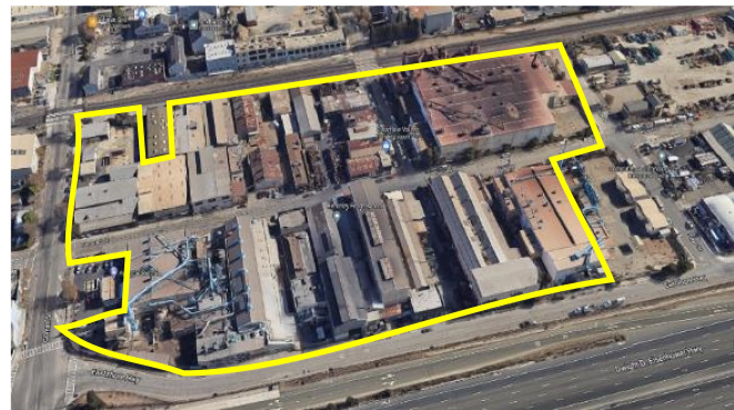
The proposed rezoning encompasses the former Pacific Steel Casting and Berkeley Forge and Tool sites, both of which have ceased operations
