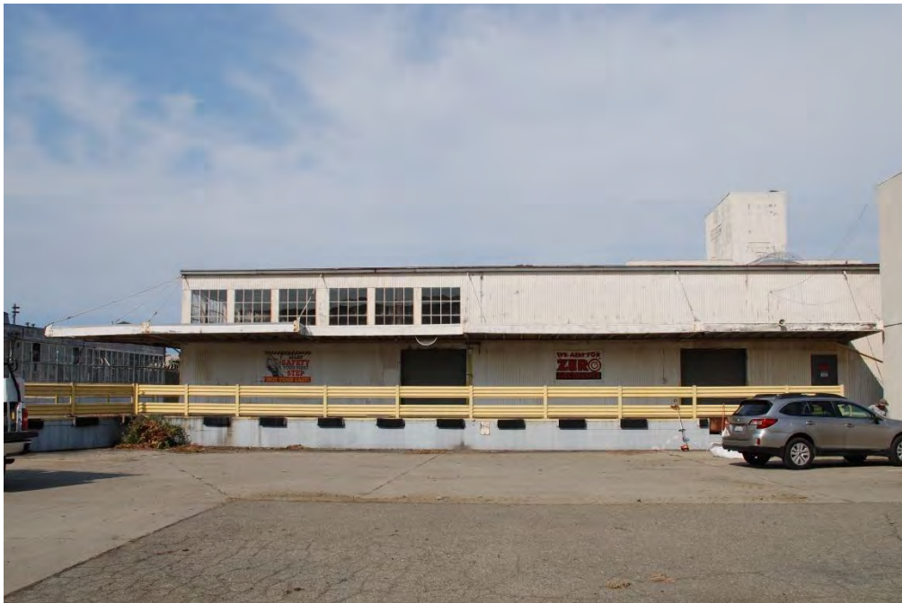
Figure 19. Warehouse and factory complex east facade, southern portion. View southwest.
