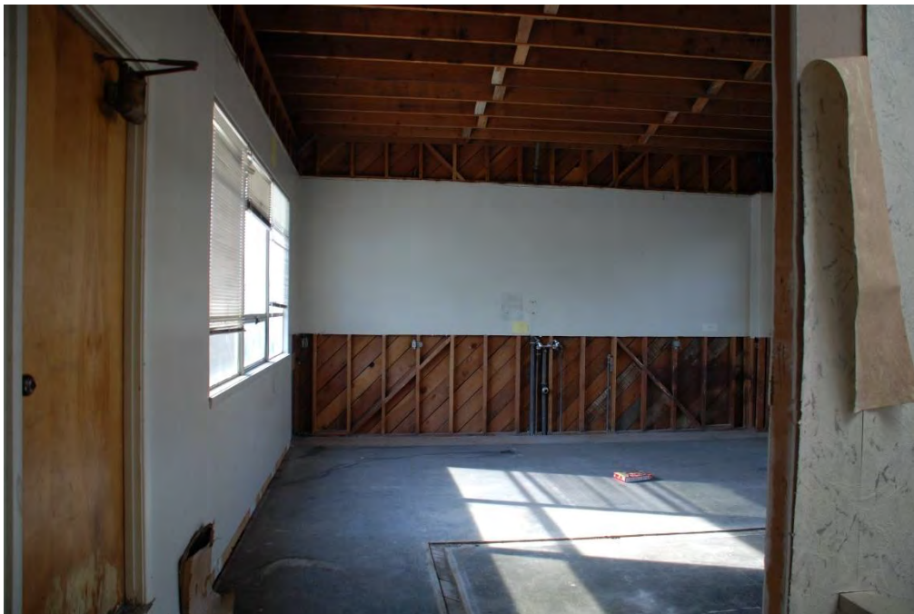
Figure 13. South space of office building second floor, view south.
