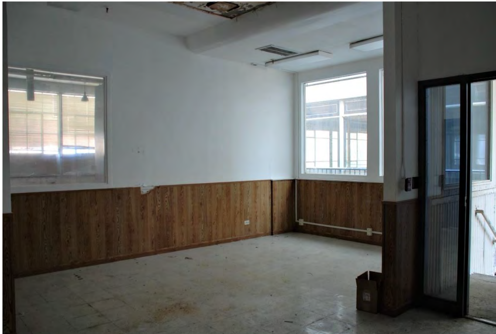
Figure 28. Entry foyer of east warehouse buildings, view northeast.
