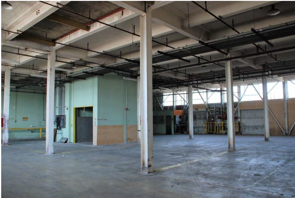
Figure 29. Central warehouse building, first floor, view northwest across main space.
