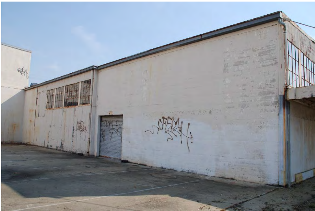
Figure 21. East warehouse building, west rear facade overlooking center of "U." View northeast.
