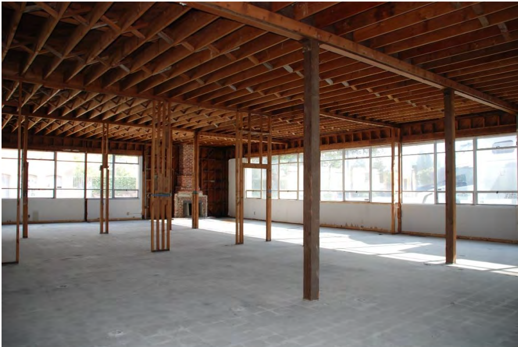
Figure 8. Office building, first floor interior, view northeast.
