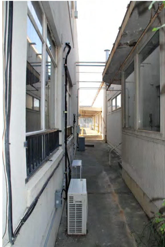
Figure 18. Warehouse and factory complex, north portion of east facade (at right of photograph), view southeast.
