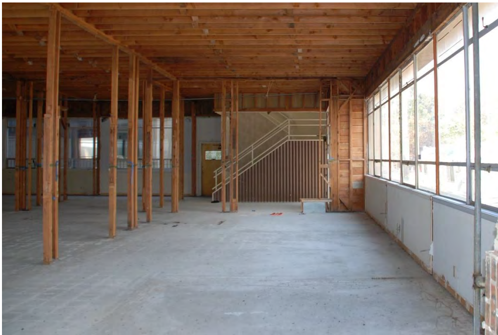
Figure 11. Staircase at northwest corner of office building, first floor, view west.
