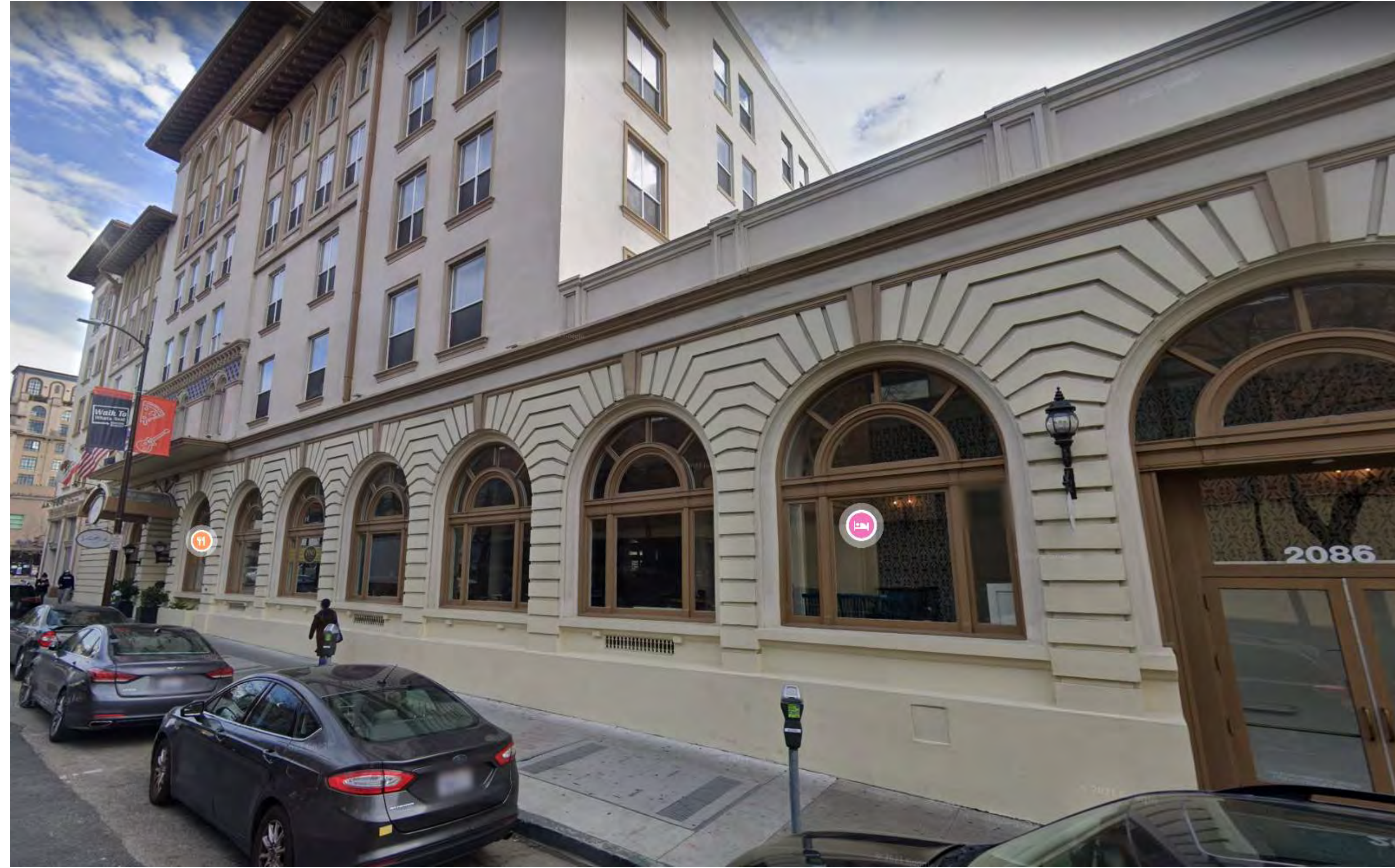
1 SITE PHOTO - ALLSTON WAY - EXISTING HOTEL A0-003 12" = 1'-0"
