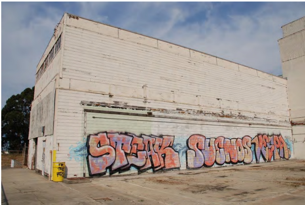
Figure 23. West warehouse building, south façade and east rear facade overlooking center of "U." View northwest.
