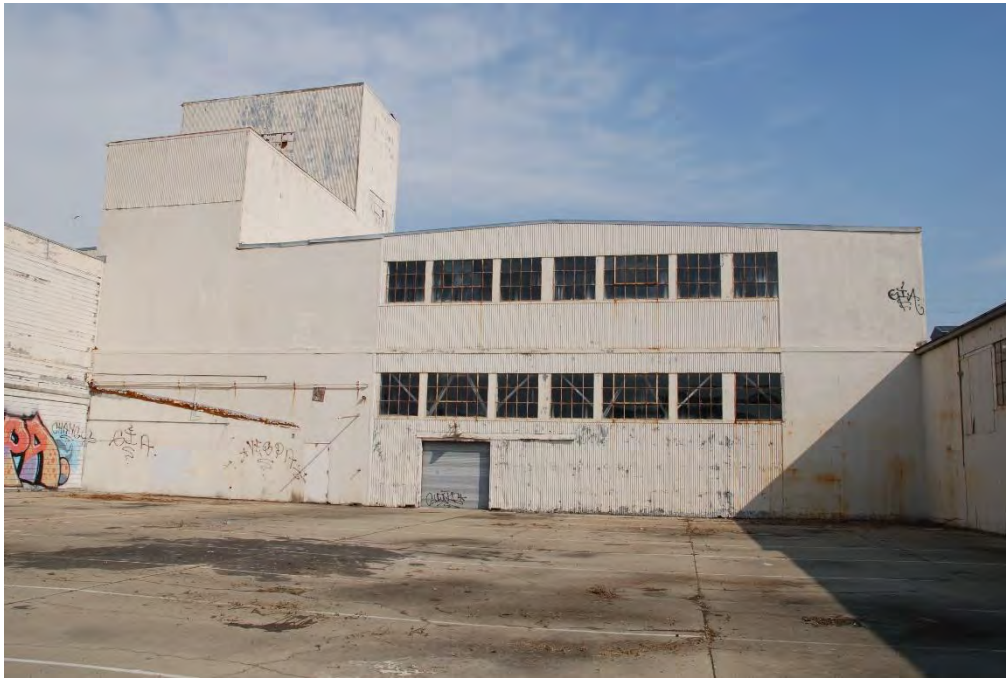
Figure 22. Central warehouse building, south facade, view north.
