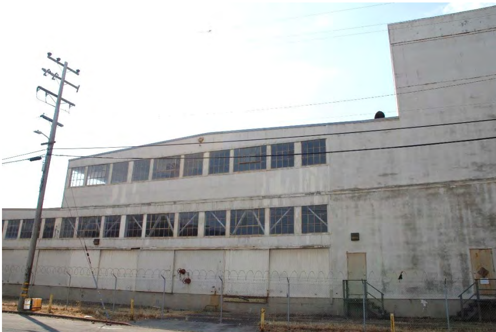
Figure 16. Warehouse and factory complex, central warehouse building, north facade. View southeast.
