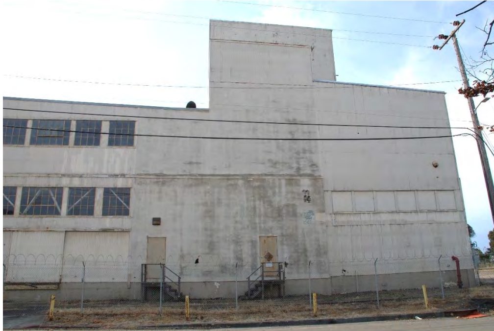
Figure 17. Warehouse and factory complex, factory building, north facade. View south.
