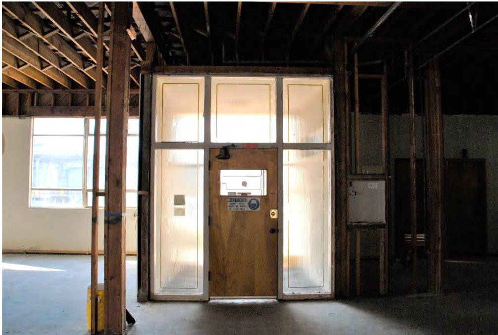
Figure 10. Office building rear entrance and vestibule, view south.
