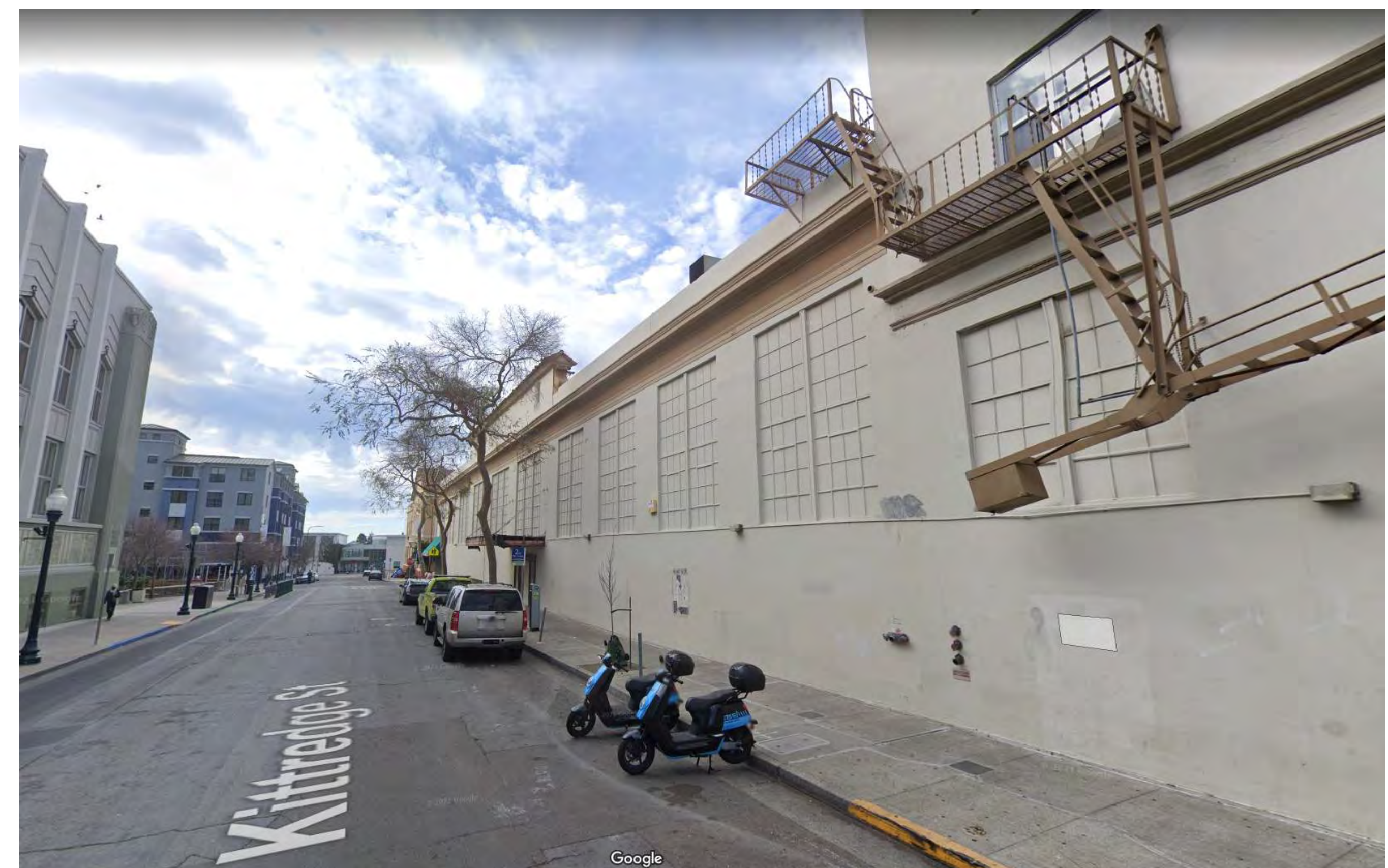
4 SITE PHOTO - KITTREDGE ST - LOOKING WEST A0-001 12" = 1'-0"
