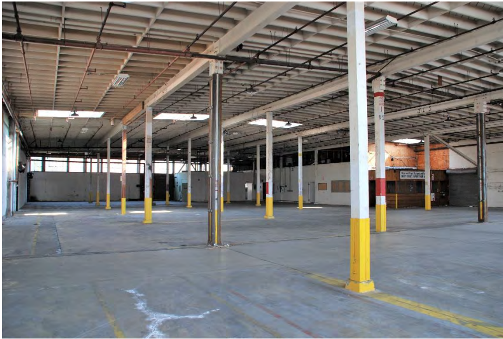
Figure 26. East warehouse building, interior of main space, view northeast.
