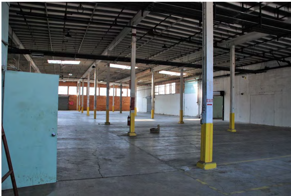
Figure 25. East warehouse building, interior of main space, view southwest.
