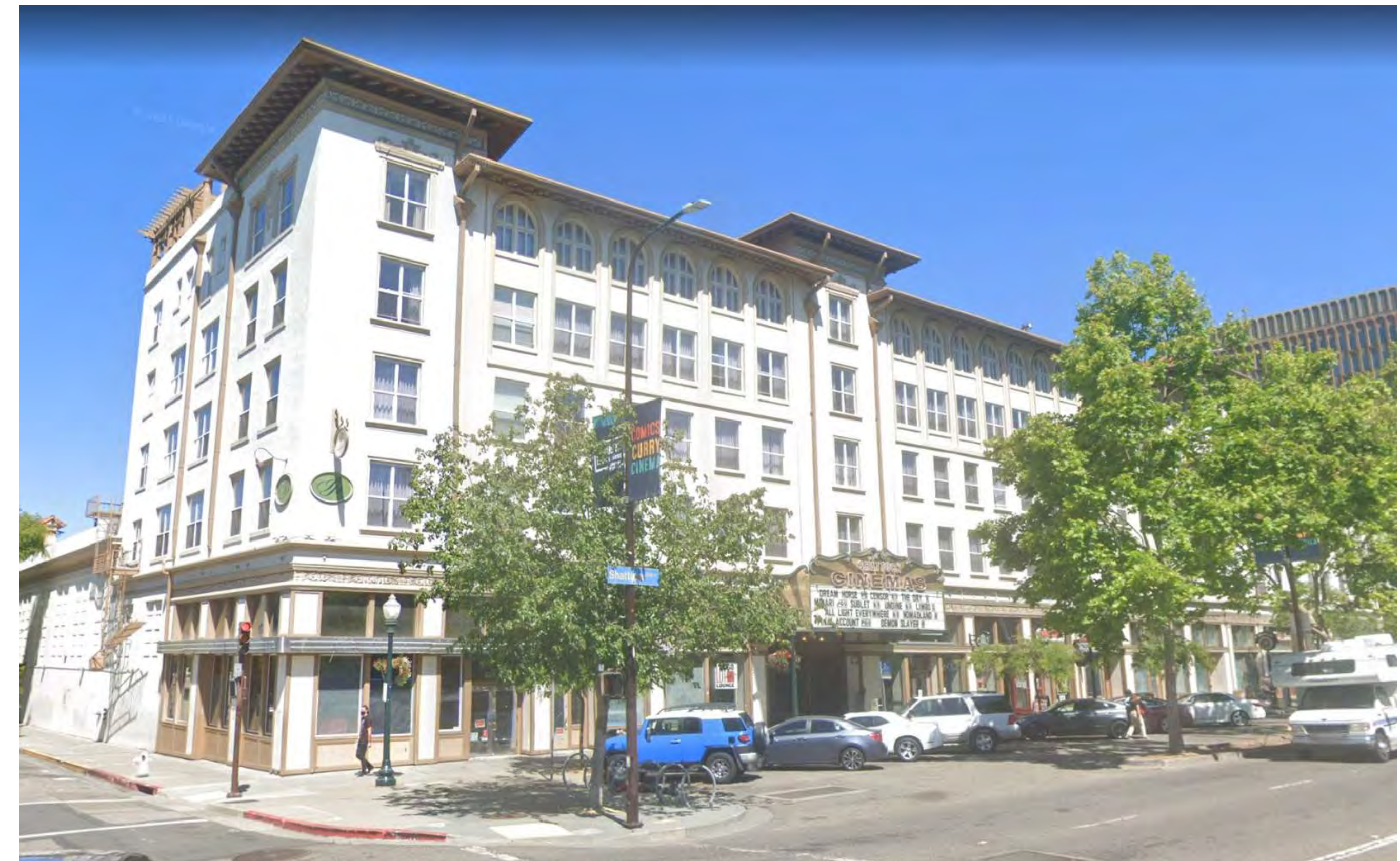
4 SITE PHOTO - SHATTUCK AVE AND KITTREDGE ST - EXISTING HOTEL A0-003 12" = 1'-0"
