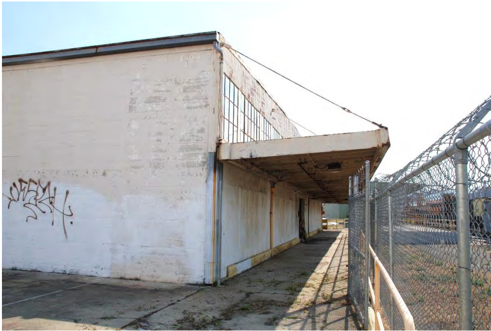
Figure 20. East warehouse building, south facade, view east.
