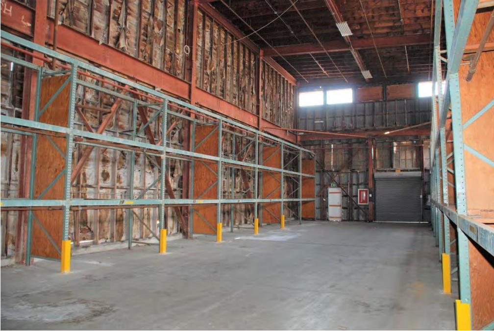
Figure 34. West warehouse building, view southeast across rear warehouse portion.
