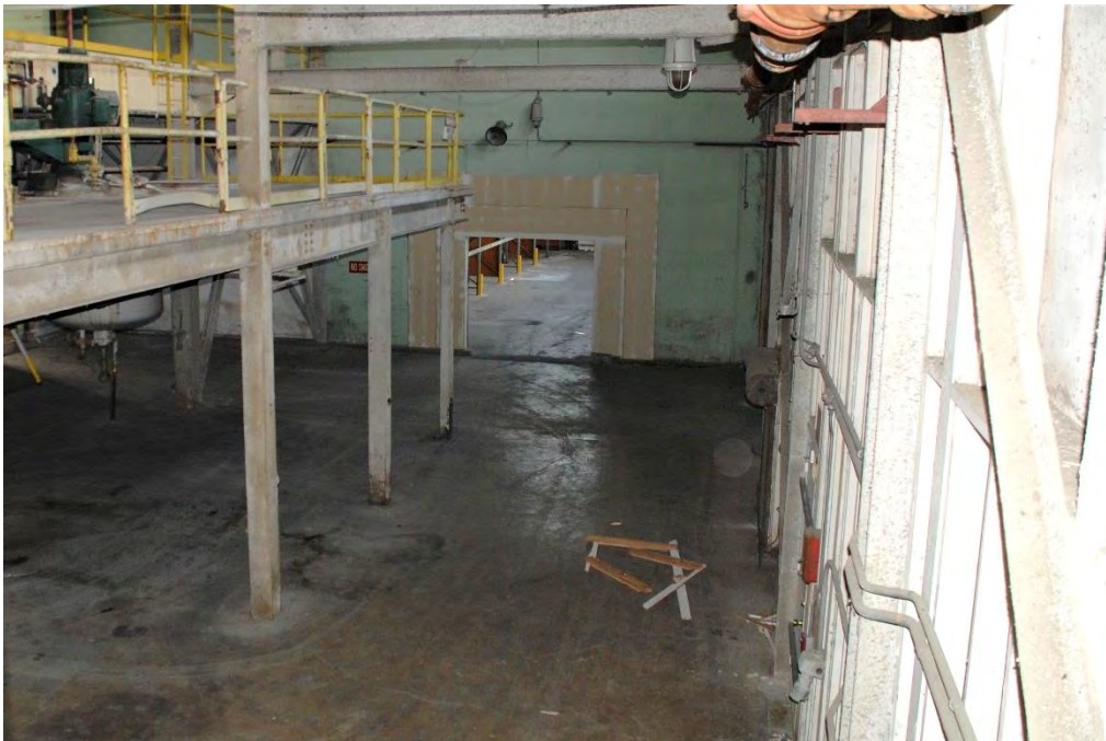
Figure 32. Factory building, view southeast from stair platform toward storage area.
