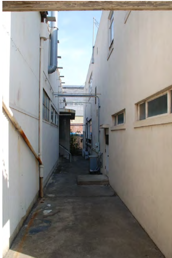
Figure 7. Office building, west facade, view north.
