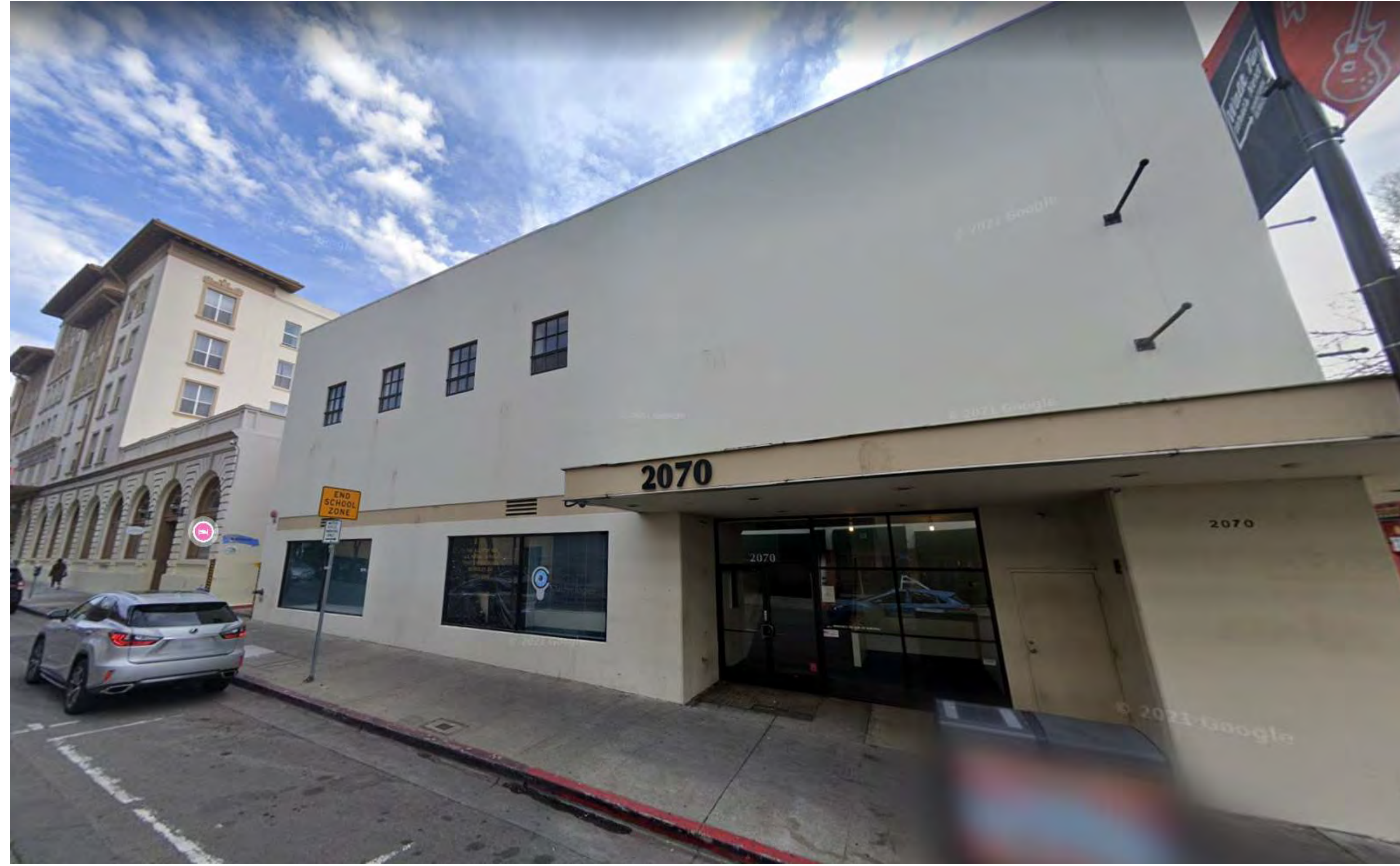
1 SITE PHOTO - ALLSTON WAY FACADE A0-002 12" = 1'-0"
