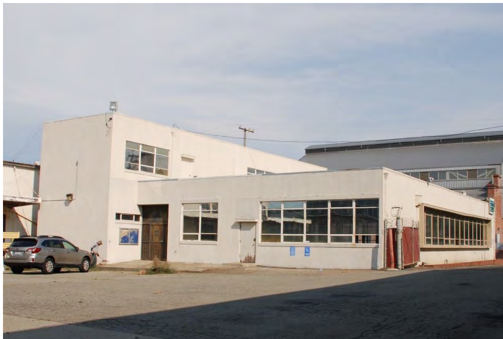
Figure 6. Office building, south and east facades, view northwest.
