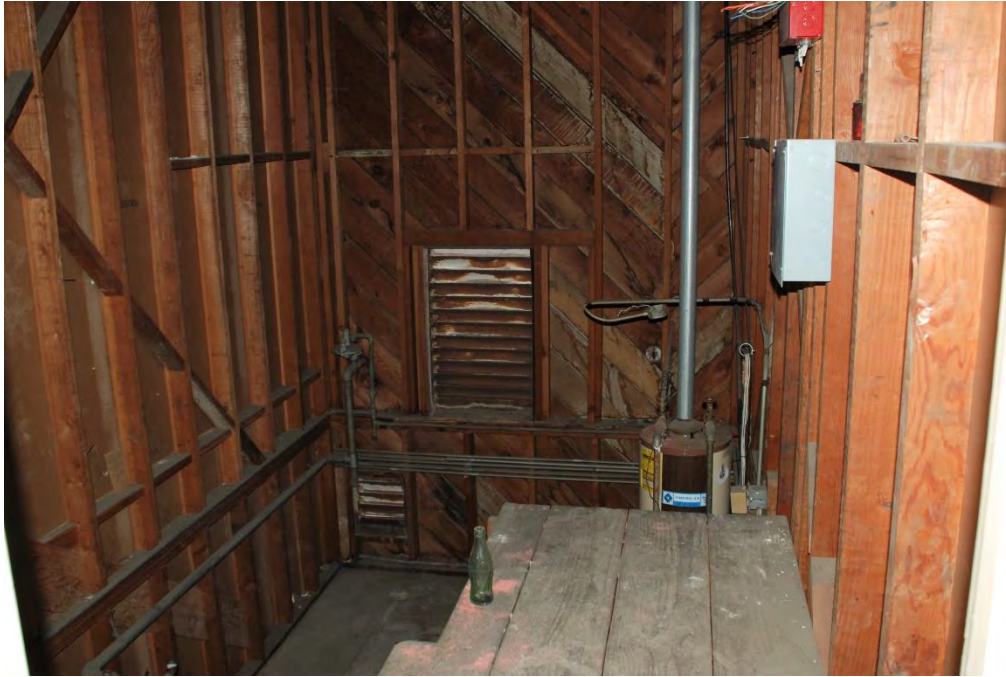
Figure 14. Second floor utility shaft, office building, view west.
