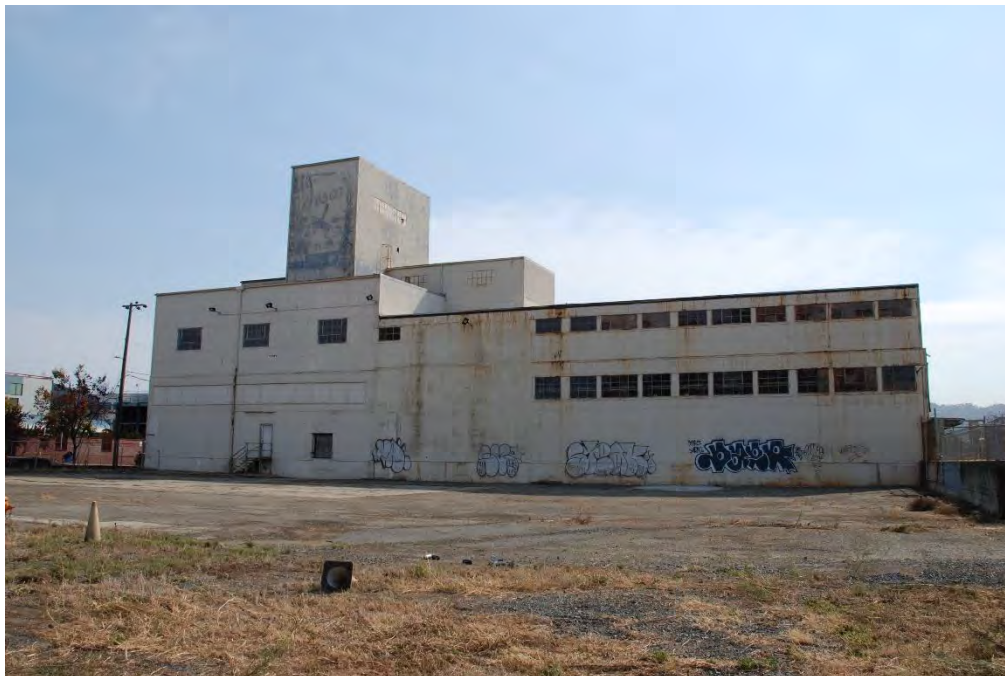
Figure 24. West facade of warehouse and factory complex. View northeast.
