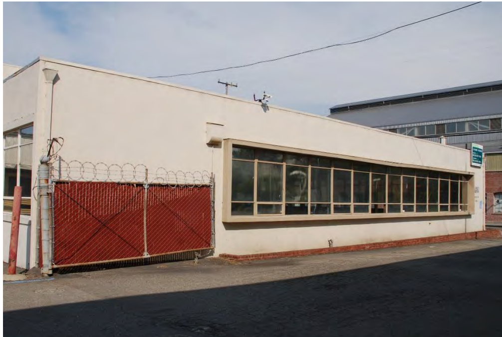
Figure 5. East Façade of office building, view northwest.
