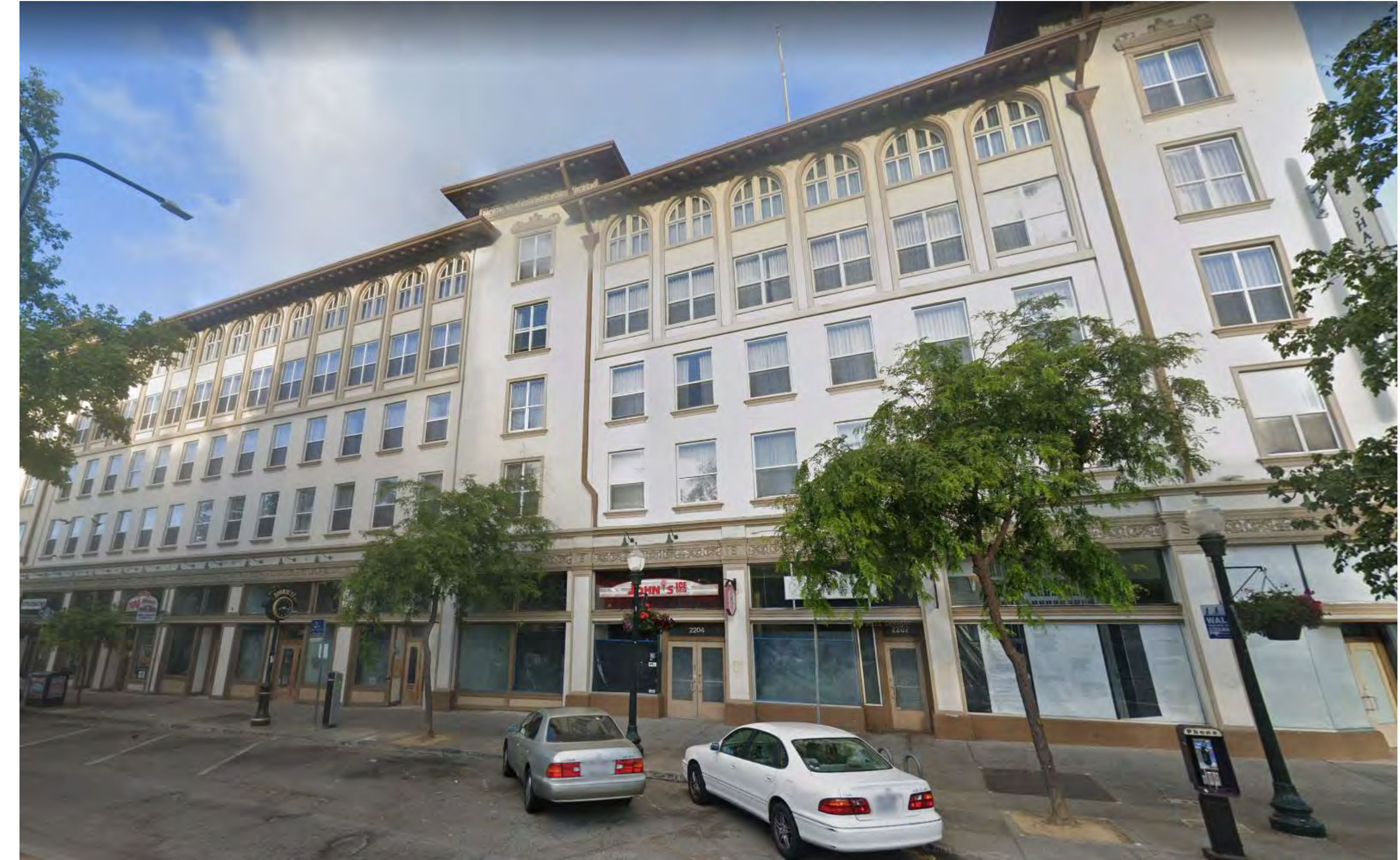
2 SITE PHOTO - SHATTUCK AVE - EXISTING HOTEL A0-003 12" = 1'-0"
