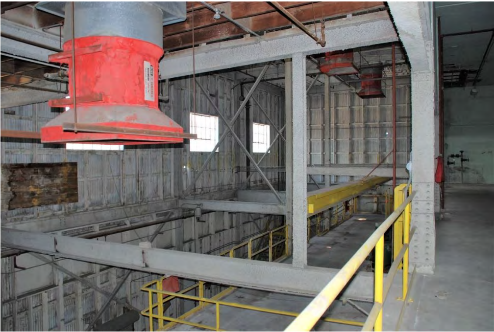
Figure 33. Factory building, view northwest from elevated platform.
