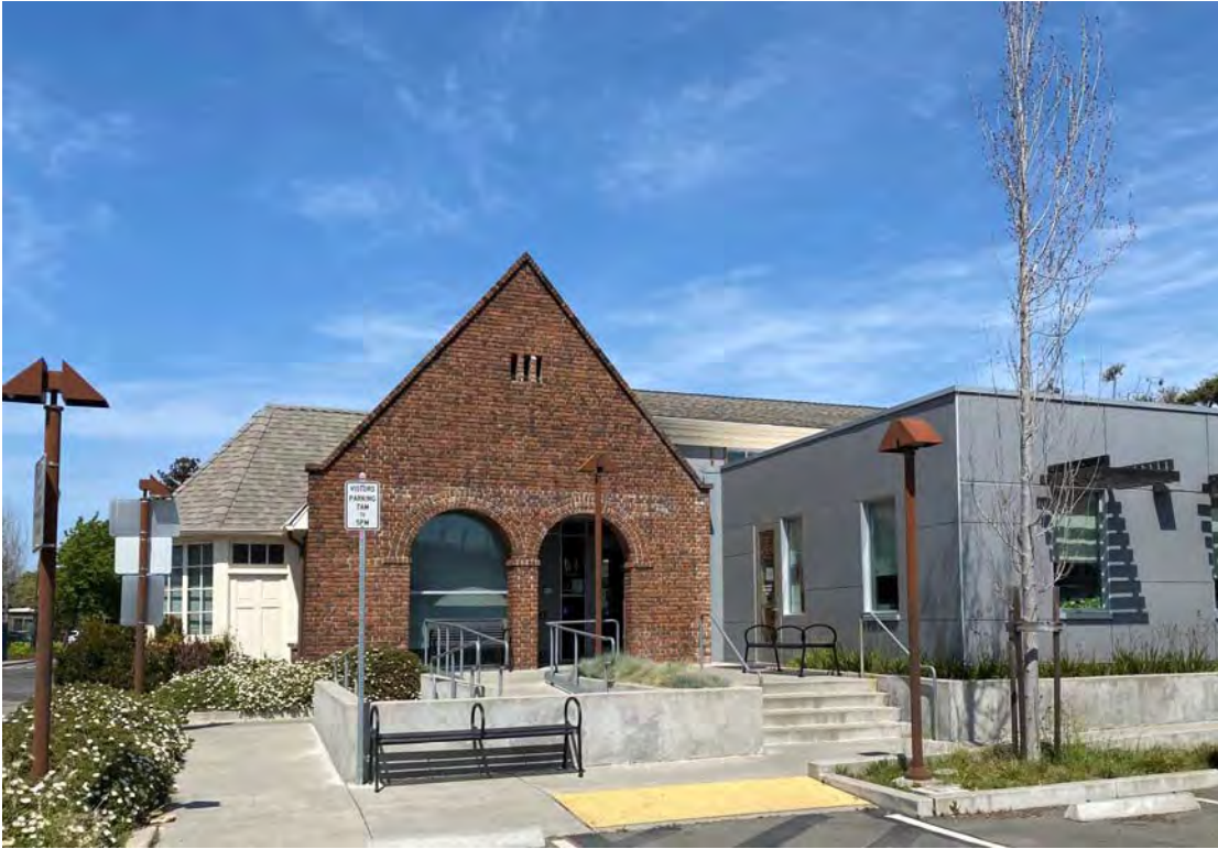
Corporation Yard Building
