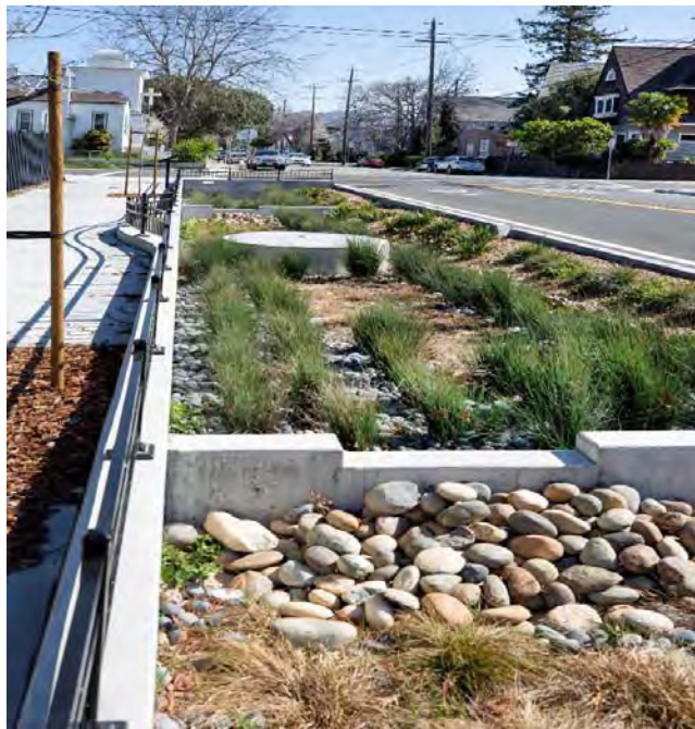
Green infrastructure installation at Woolsey Street
