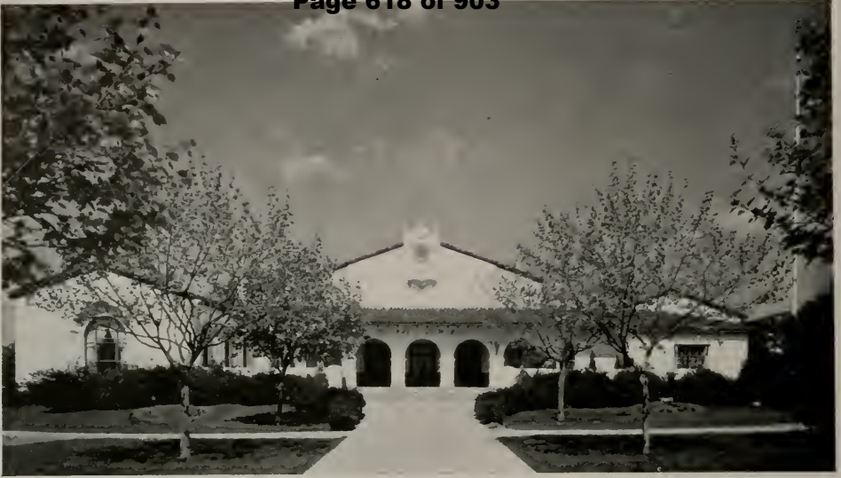
VETERANS MEMORIAL BUILDING, ALBANY, CALIFORNIA Henry H. Meyers, Architect George R. Klinkhardt and Mildred S. Meyers, Associate Architects
