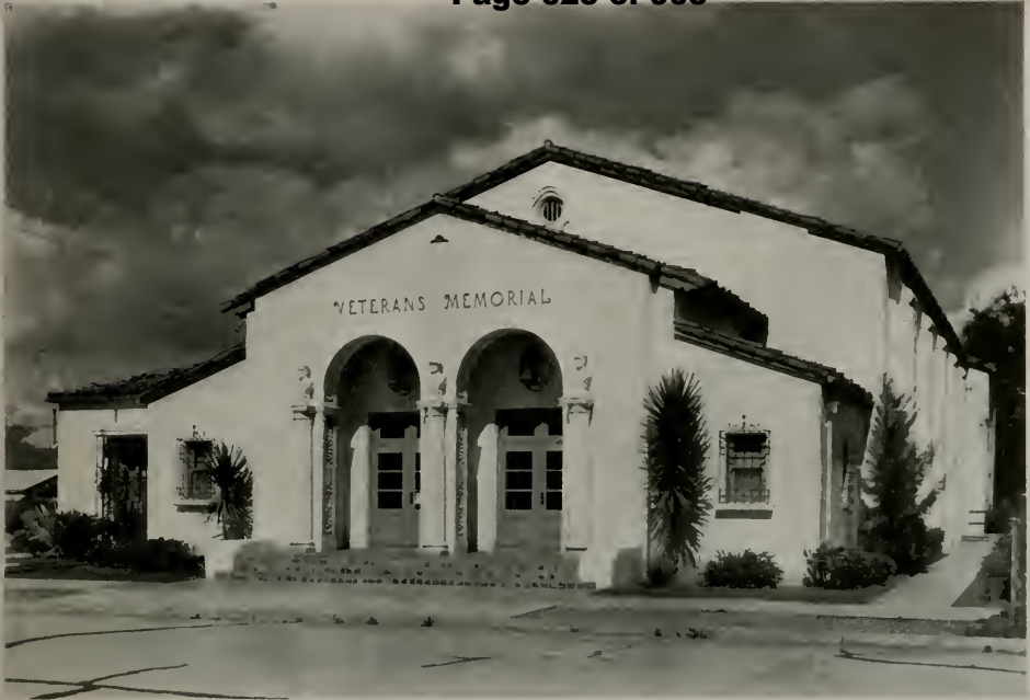
VETERANS MEMORIAL BUILDING, LIVERMORE, CALIFORNIA Henry H. Meyers, Architect George R. Klinkhardt and Mildred S. Meyers, Associate Architects
