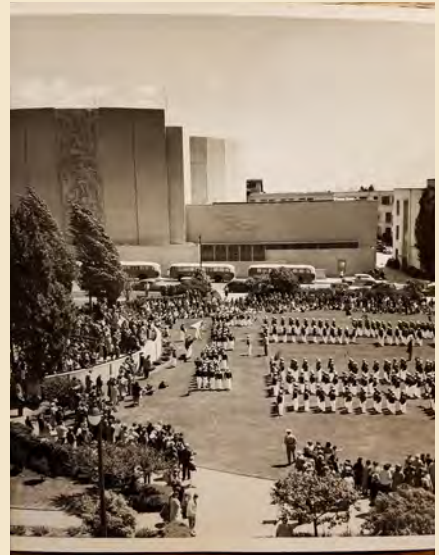
Figure 4.23 The south side of the Berkeley High School Community Theater, designed by Gutterson and Corlett Architects, and Civic Center Park with some established plantings, 1951. Source: Berkeley History Collection, Berkeley Public Library.
