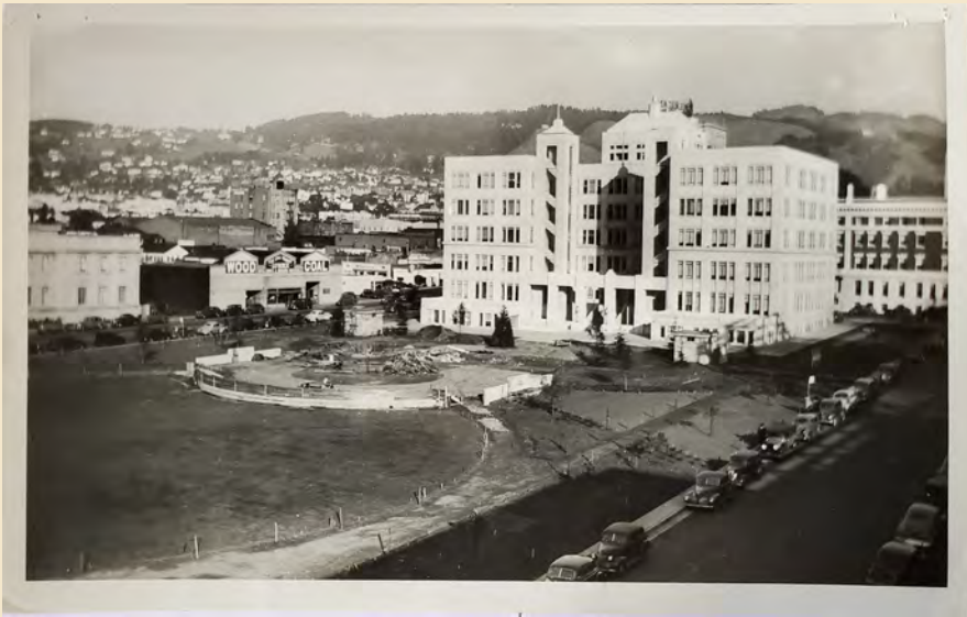
Figure 4.19 Federal Land Bank Building with the Civic Center Park fountain under construction, 1941-42. Source: Berkeley Architectural Heritage Association.
