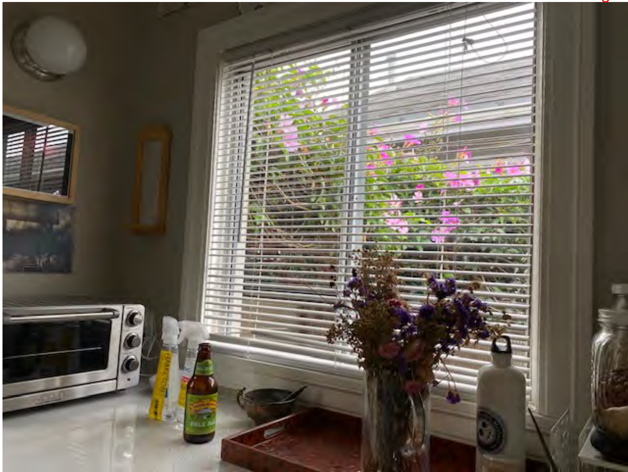
You can see the current roof line through the kitchen window. I took the picture today, with an overcast sky, so it is difficult to see.
