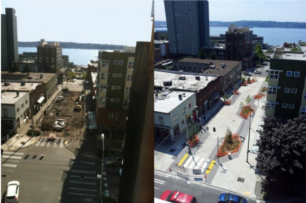
Bell Street, during and shortly after construction.
