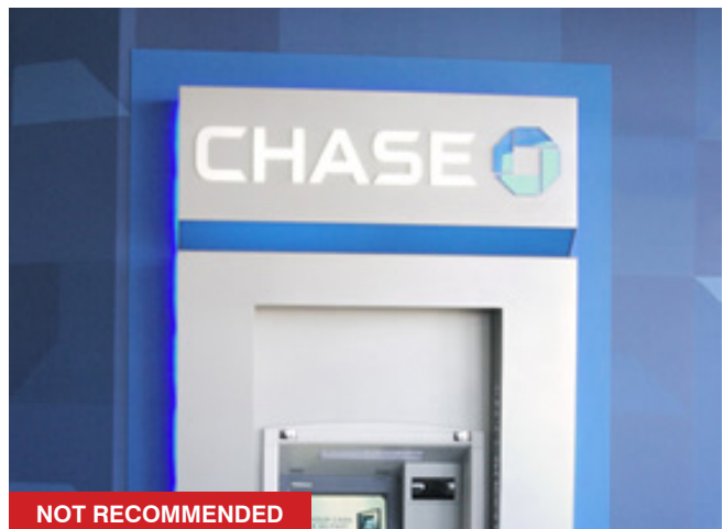
Colorwashing a building facade in branded color serves as oversized signage and is not permitted.
