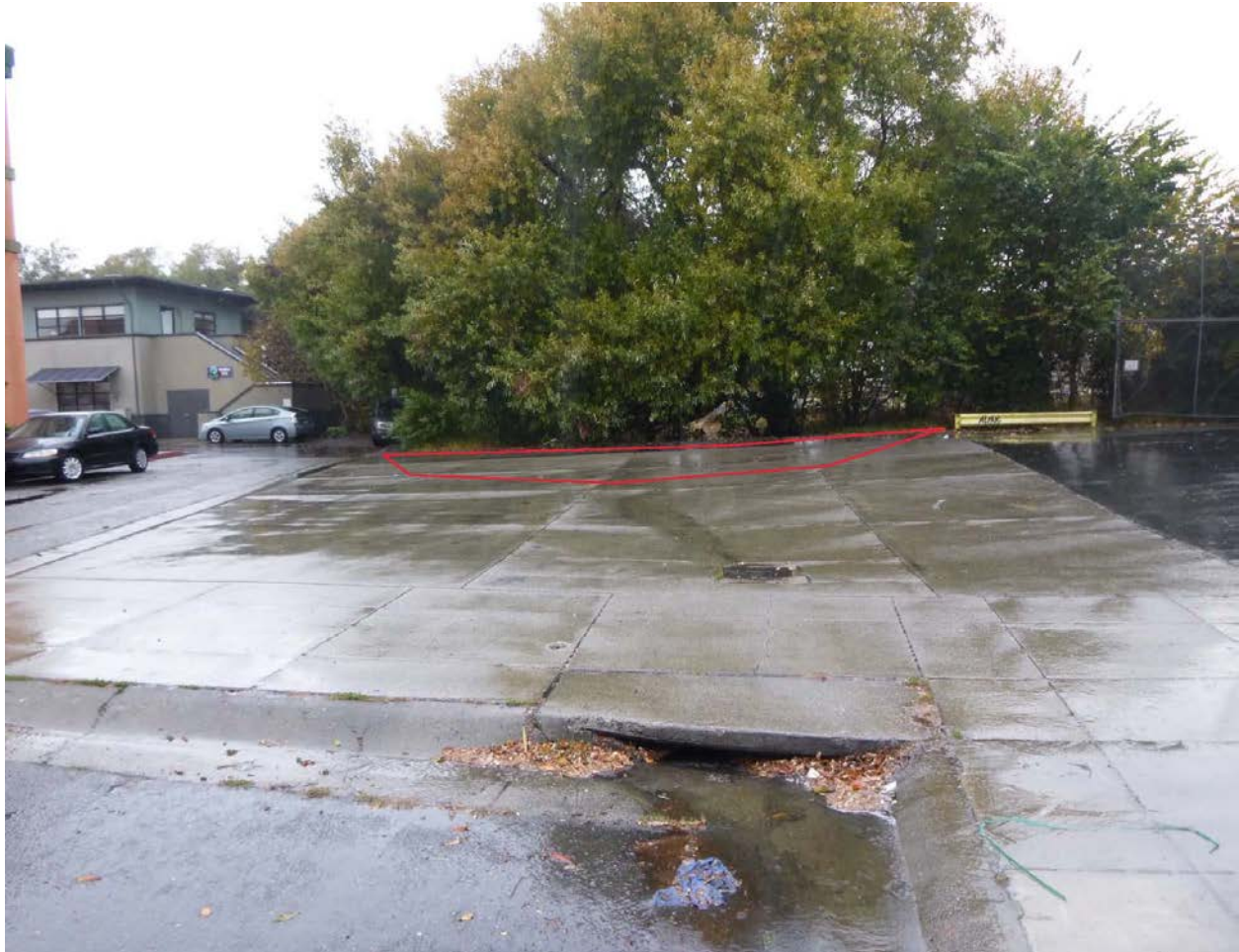
Figure 16 – A portion of the raised concrete surface on Ninth Street at Codornices Creek could be converted into a bioretention feature.
