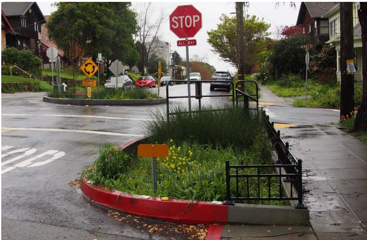
Figure 7 – Connected bioretention features in a traffic circle and corner bulb-out at Spruce and Vine Streets.
