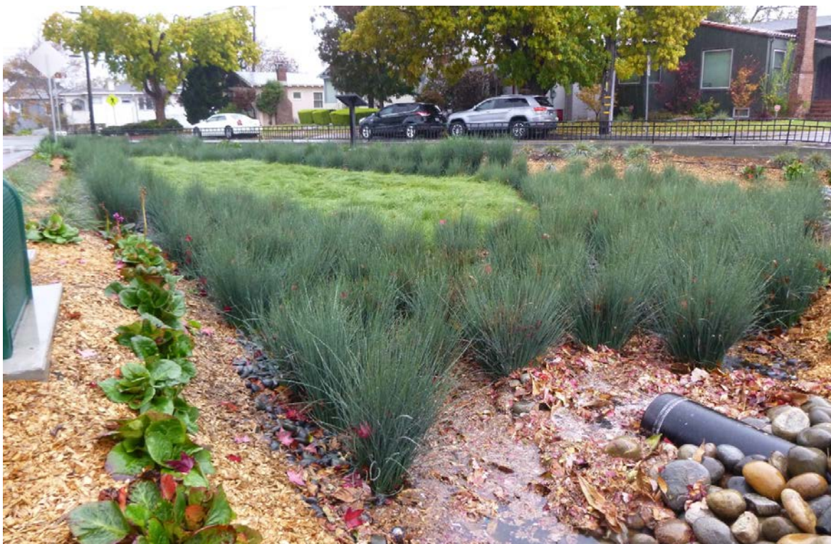
Figure 5 – A large concrete traffic island/median was reconstructed with a bioretention facility at Rose and Hopkins Streets.
