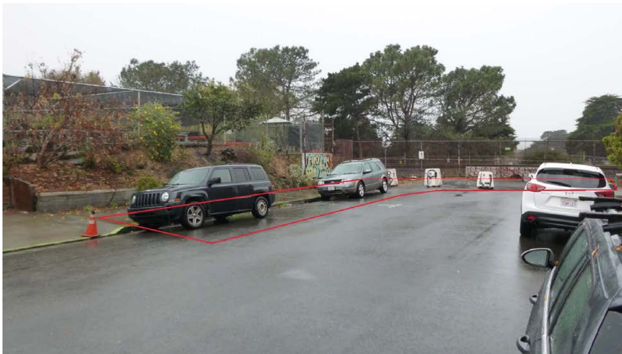
Figure 27 – Potential Location for a Bioretention Feature on Channing Way at the UPRR ROW
