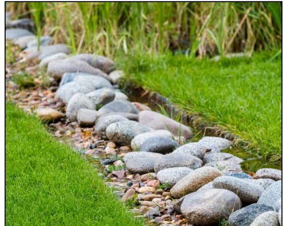
Figure C-8. Pervious Drainage Channel. Pervious, unlined drainage channels can be designed to convey runoff to GI facilities.
