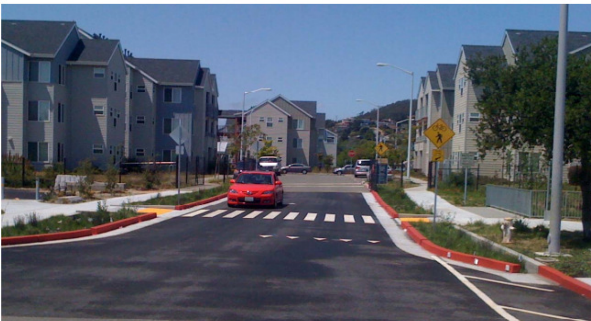
Figure 18 – Existing bioretention features on Sixth Street that treat runoff from the street prior to running into the creek show how similar treatment at Tenth Street could be implemented.
