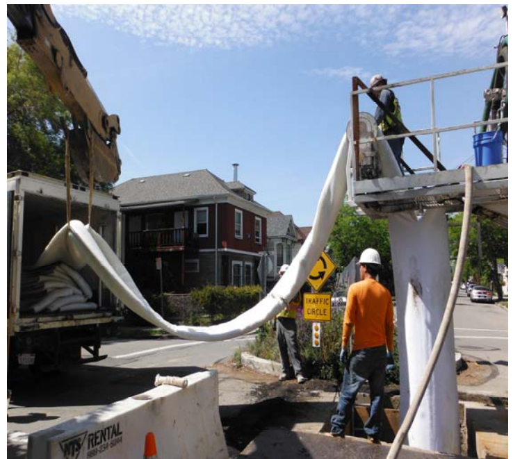
Woolsey Street Sanitary Sewer Rehabilitation
