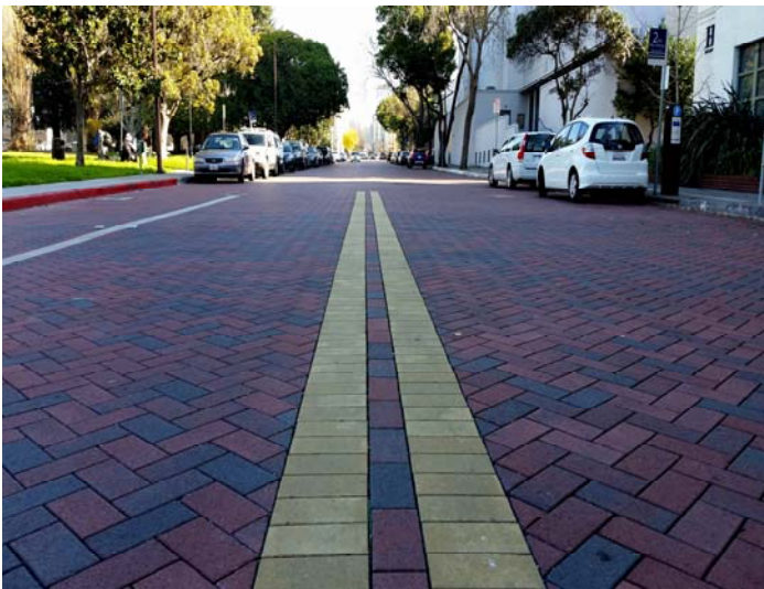
Allston Way Permeable Pavers
